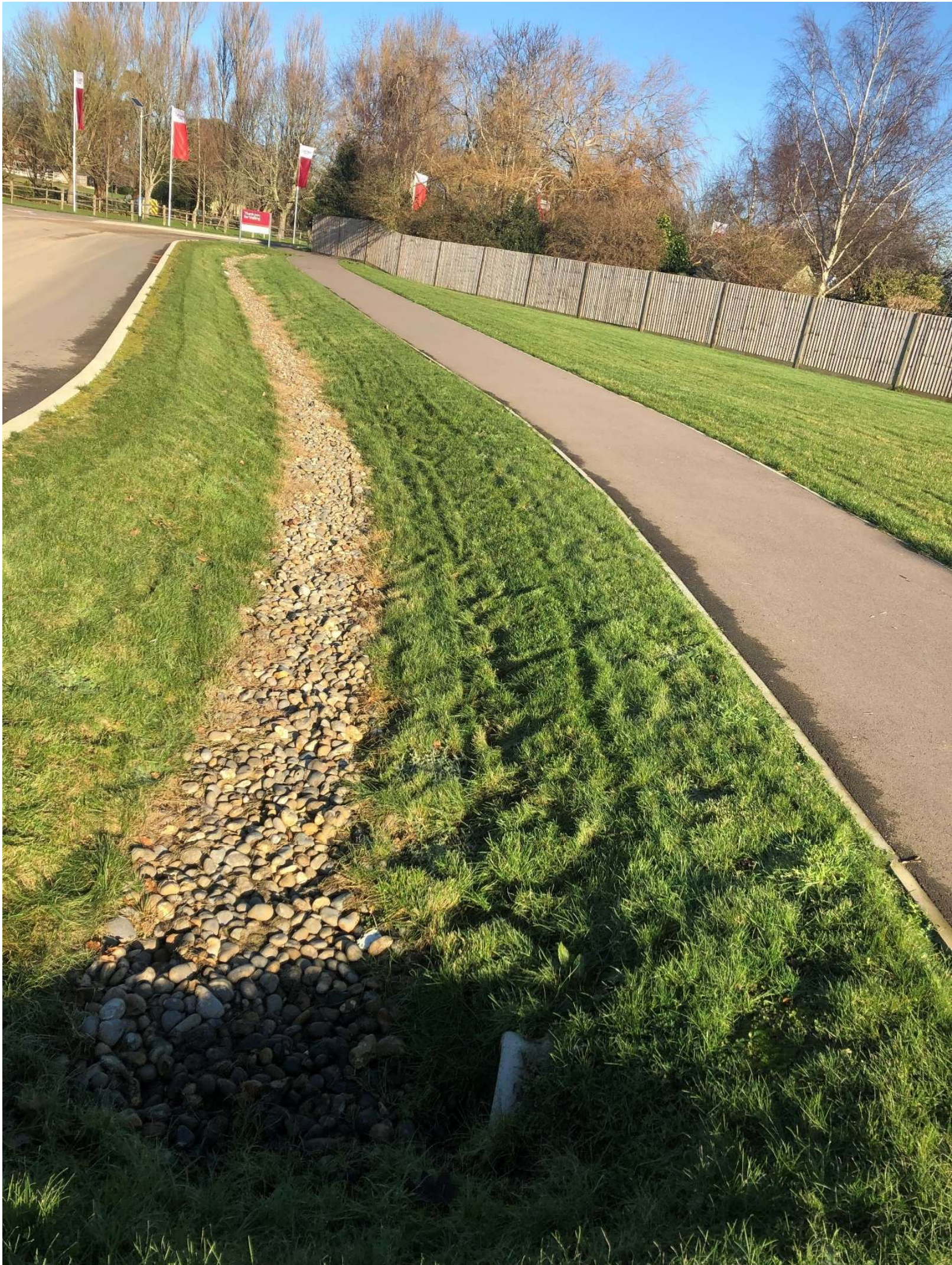
Swale E - 17 January 2022 - complete and functioning
