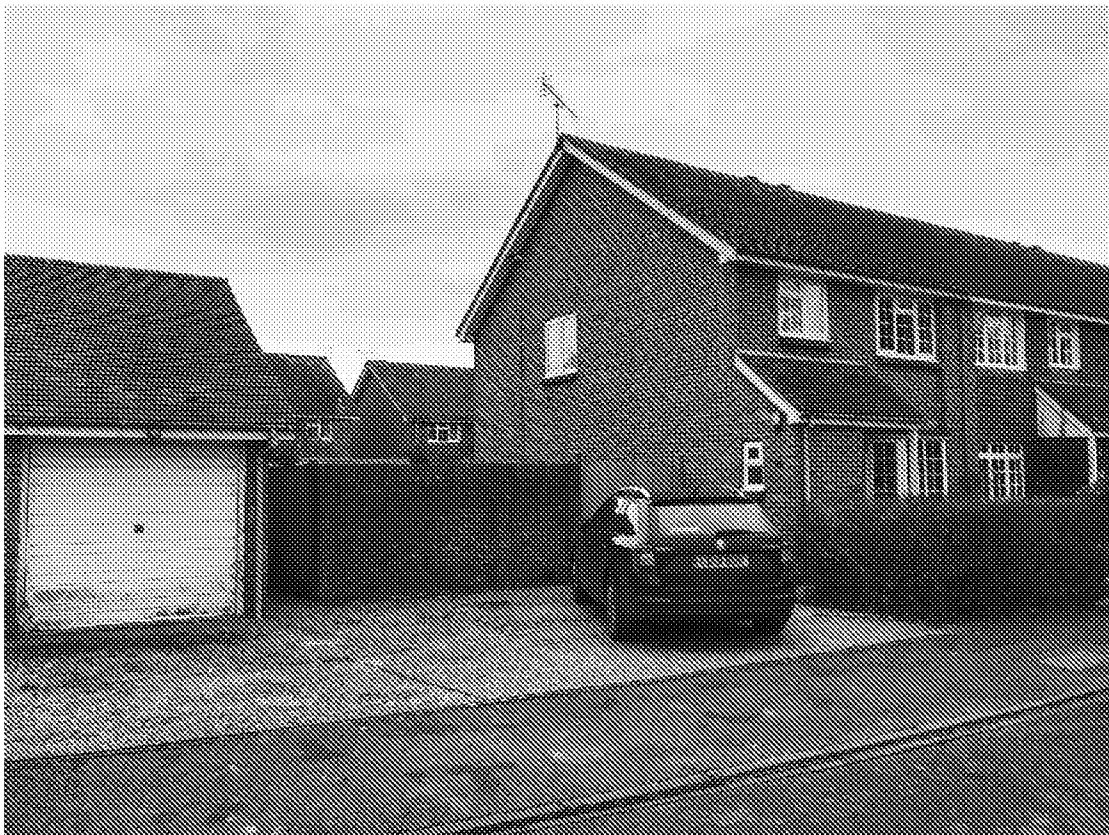
Fig 1. The proposed site, with communal access and garages adjacent to east
