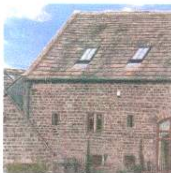
Centre-pivot and top-hung windows.
