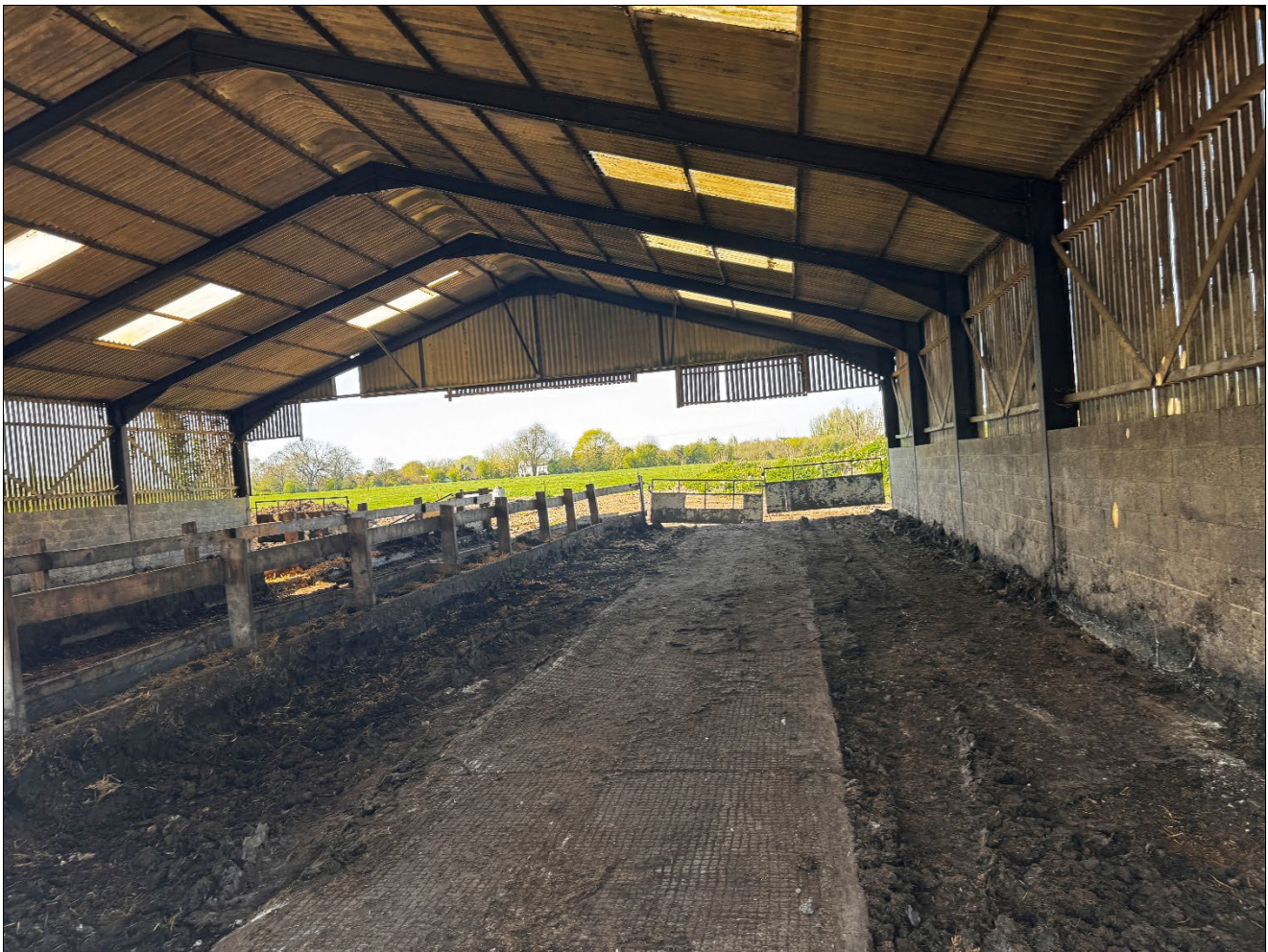
Figure 11 Internals of plot 4,5,6 with steel frames
