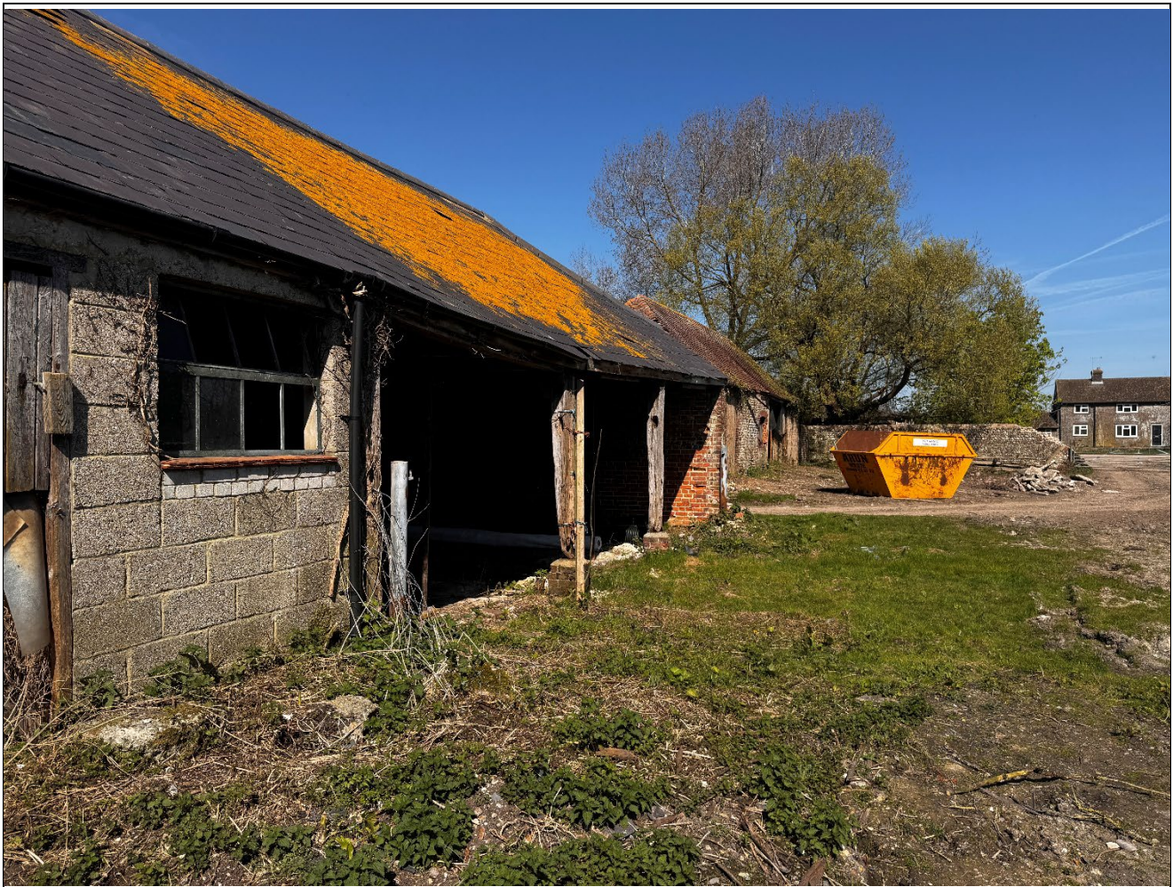
Figure 13 Plot 8 East elevation to cart shed with infill blockwork walls
