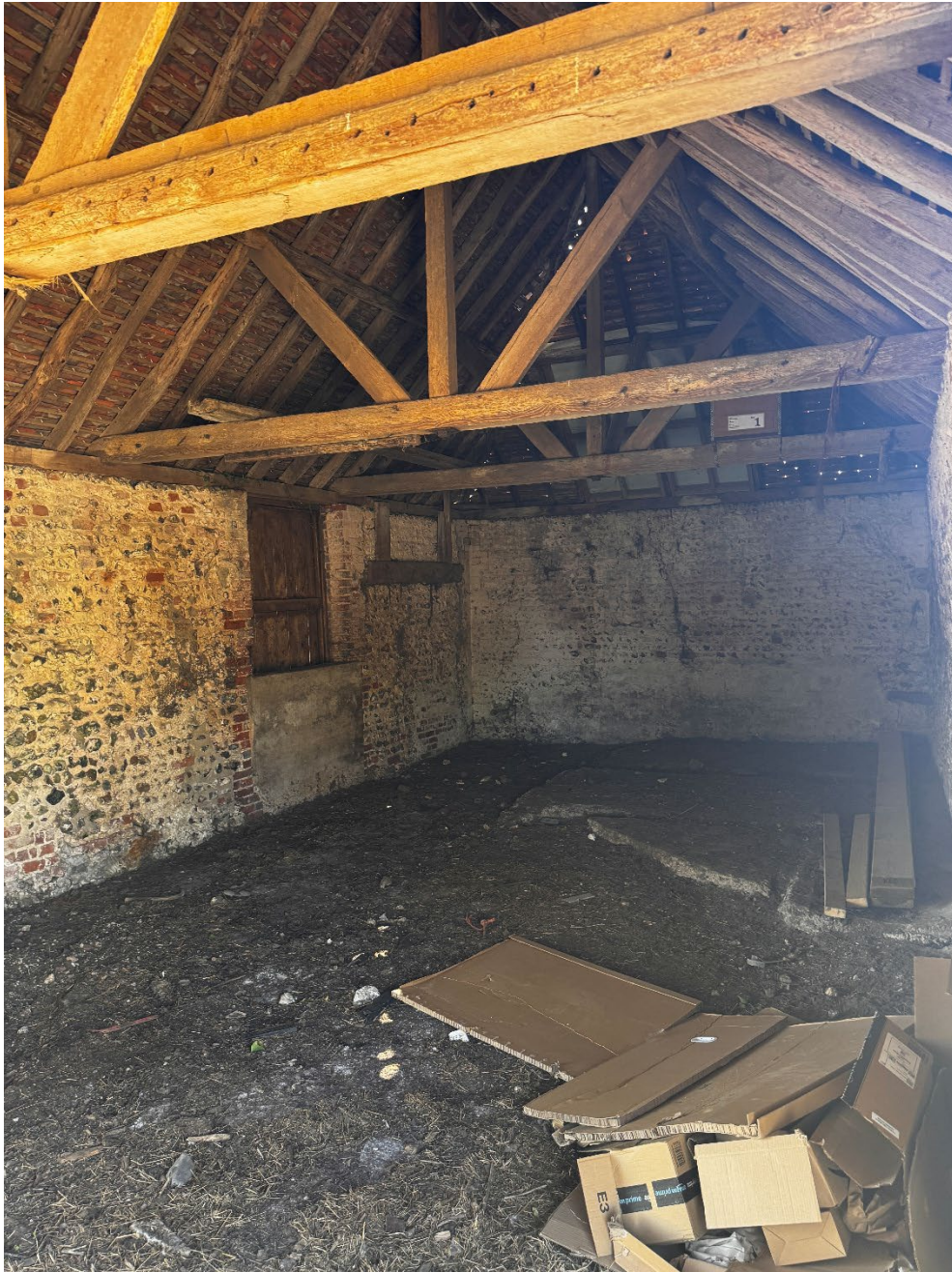
Figure 9 roof structure of plot 9
