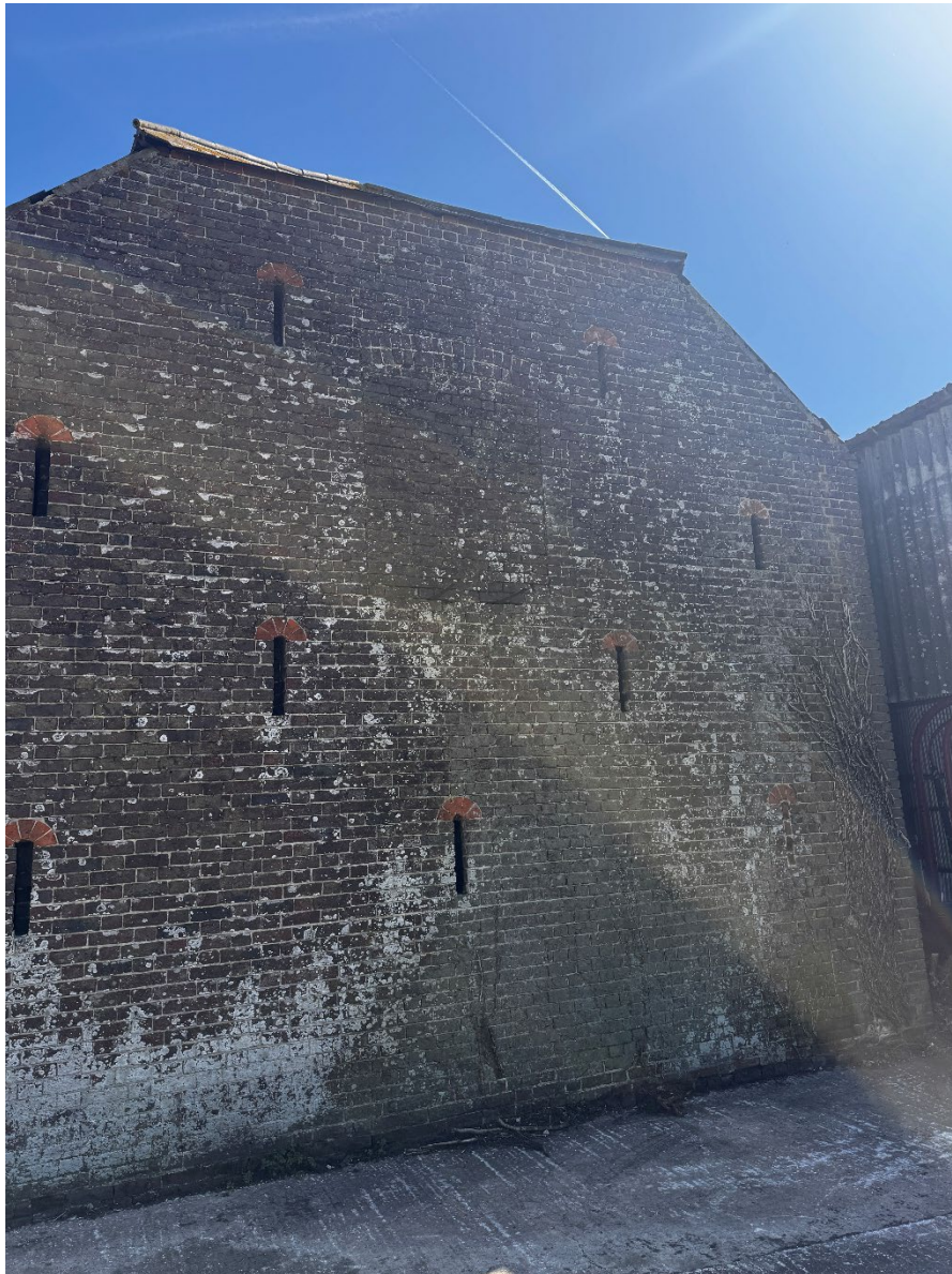
Figure 4 Gable Wall of Plot 2 with plot 3 in the right side.
