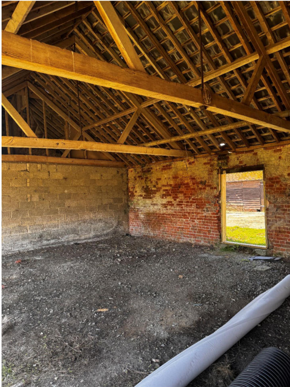
Figure 14 internal roof structure of Plot 8
