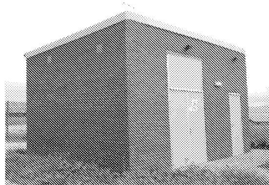
DNO Substation, Little Trevease Cornwall
