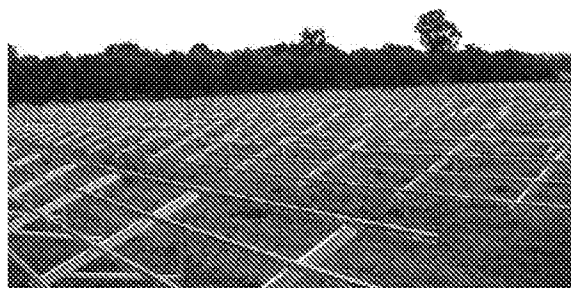
Frame structures prior to attachment of panels
