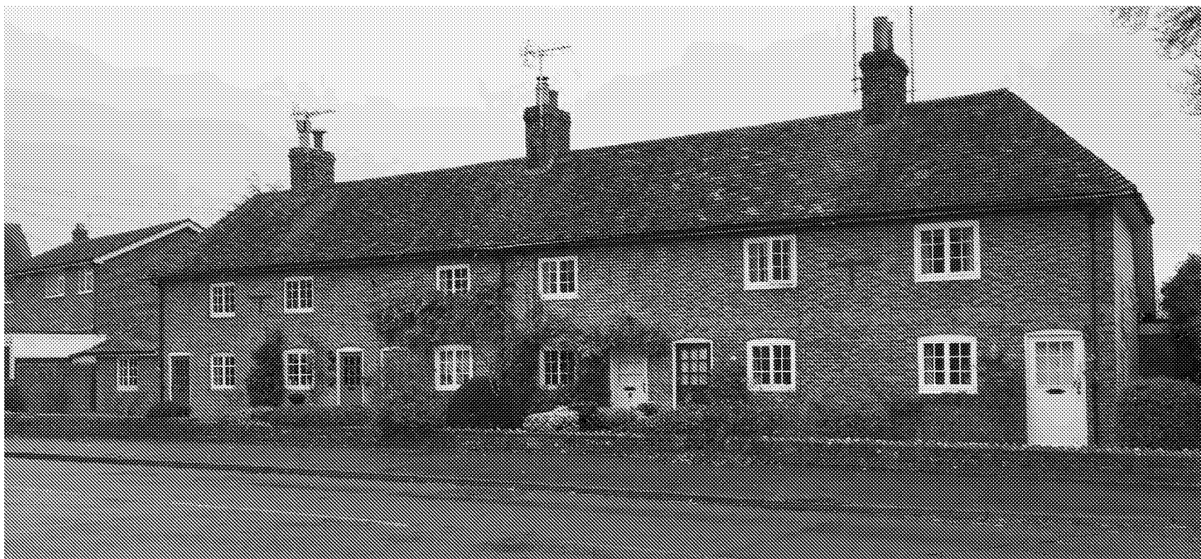
Plate 31: Nos. 15–20 The Street, principal northern elevation.
