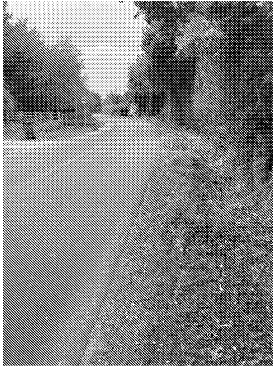
Photograph 1: Eastergate Lane Existing Conditions
