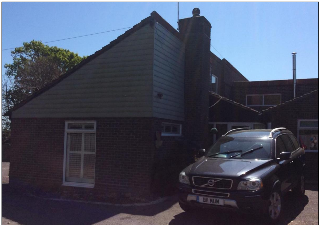
Photograph 12. Mix of brick and weatherboarding walls on the northern face of the property.
