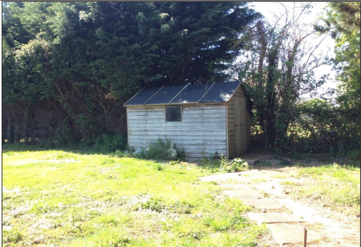
Photograph 11. View westwards of the small shed situated on the western site boundary.
