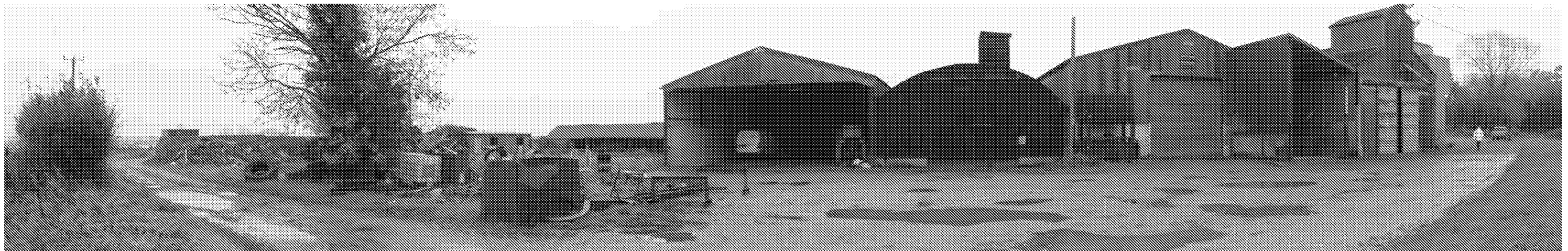
Photograph C. South eastern view adjacent to a series of poor condition and quality agricultural buildings including a grain store, adjacent to the earlier farmstead, (to left of view) .
