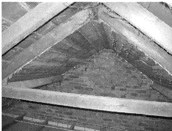
Timber on rafters at eastern end
