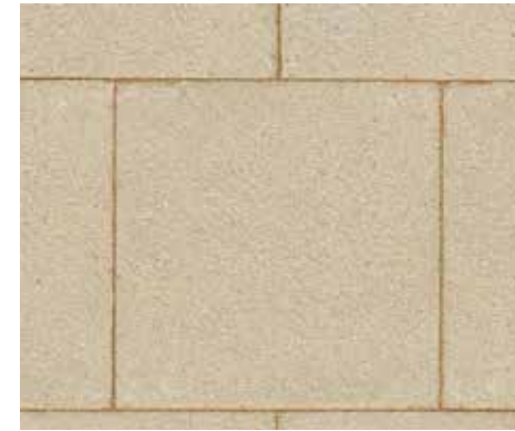
Natural tone concrete paving slabs to shared pedestrian pathways and patios.
