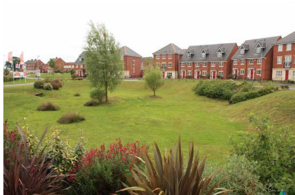
Planted attenuation basin
