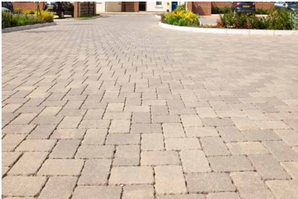
Permeable block paving of a natural tone to shared driveways.
