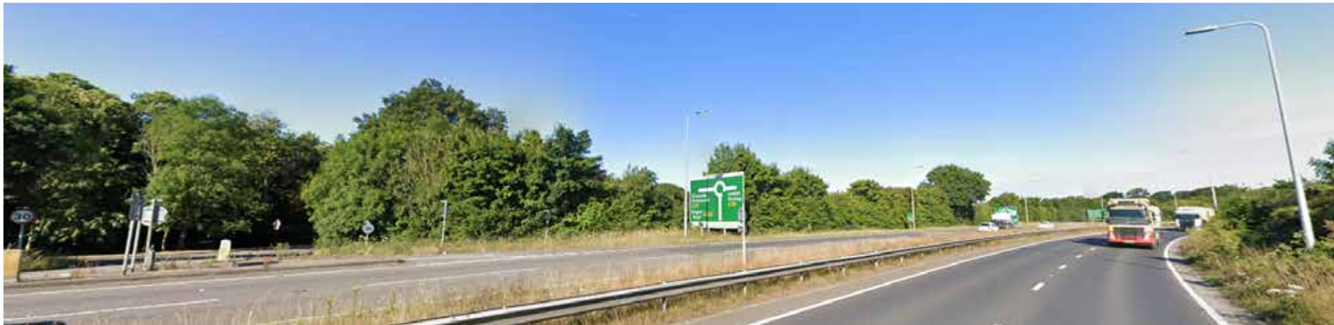
Photograph A - View, looking west, of the northeastern vegetated Site boundary, from the from the east-bound side of the A27. To the left is the turn-off onto Arundel Road.
