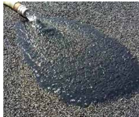
Permeable asphalt to main vehicular access road.
