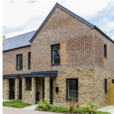
Projecting header course defining entrances and replicating flintish bond detail on building edges
