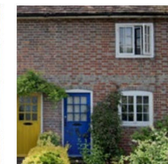
Horizontal brick banding
