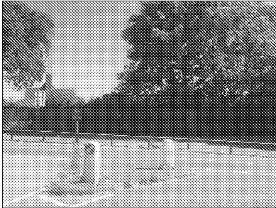
Figure 4. Fence-line looking South onto application site from Dukes Road
