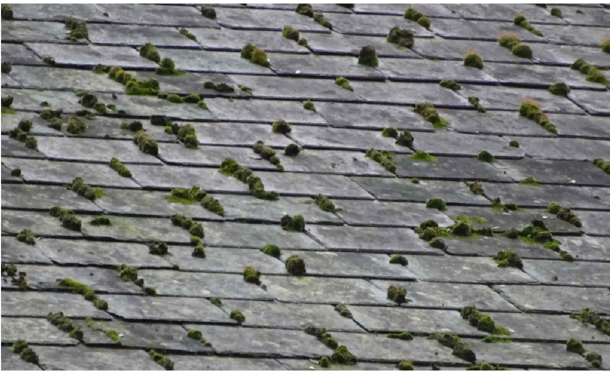
Photo of Existing Roof Tiles (N.T.S)
