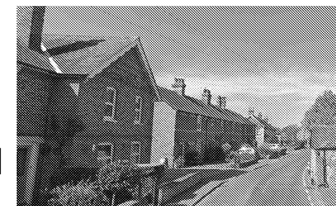
2. High Street looking North
