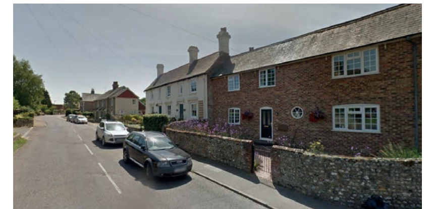
5. High Street looking South
