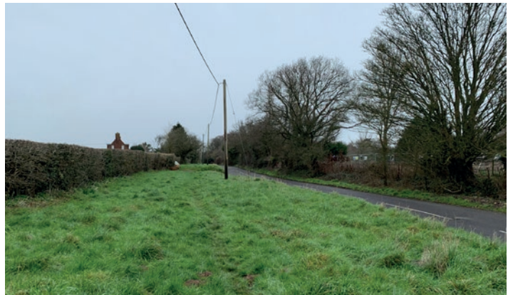
1. Tye lane looking north
