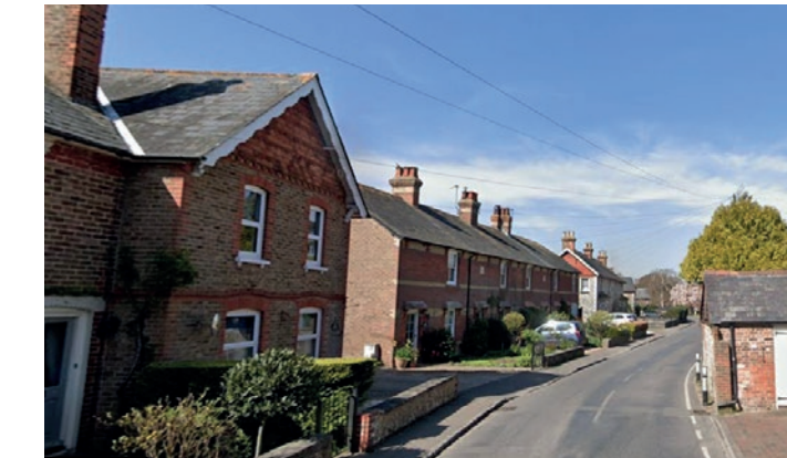
2. High Street looking North
