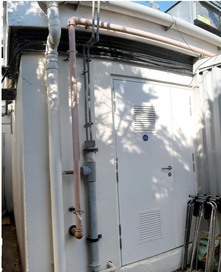
Figure 6 – Existing Plant Room
