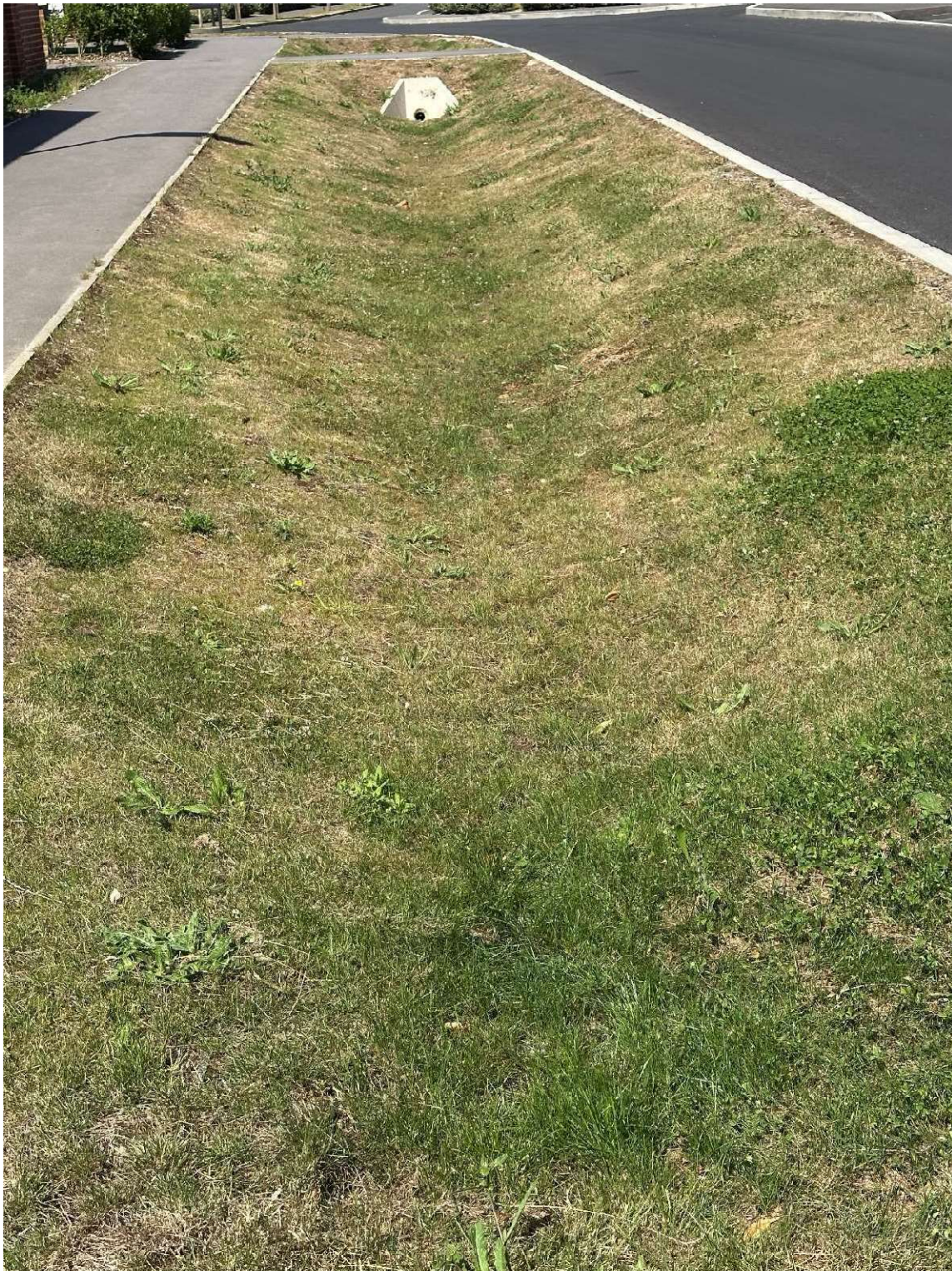
Swale U – 16 th July 2025 - complete and functioning
