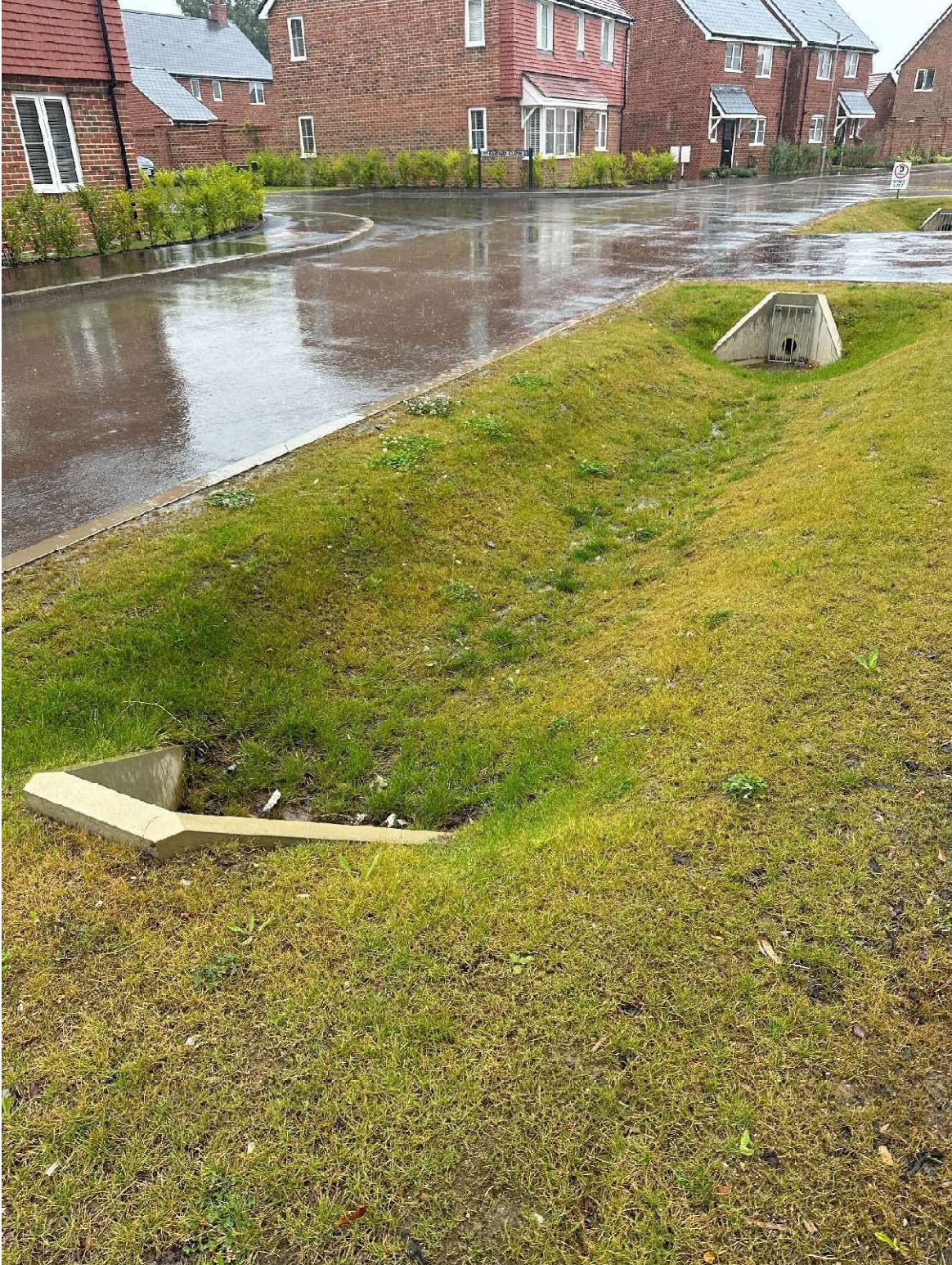
Swale P-Q-HW2C-G - 9 July 2024 - complete and functioning
