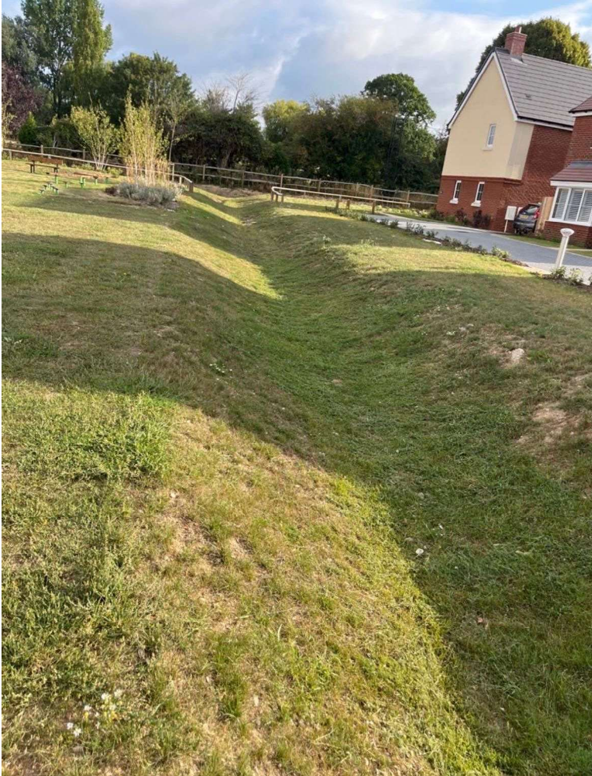
Swale B (Spur) – 16 th July 2025 - complete and functioning
