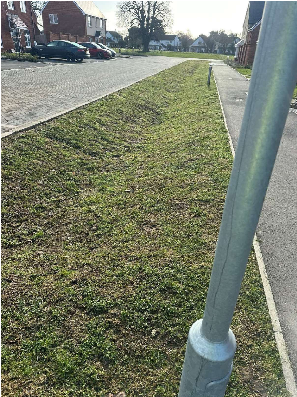
Swale I - 01 February 2023 – complete and functioning
