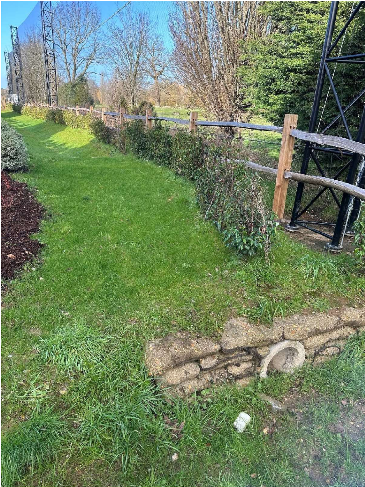
Head Wall 1B - 01 February 2023 - complete and functioning
