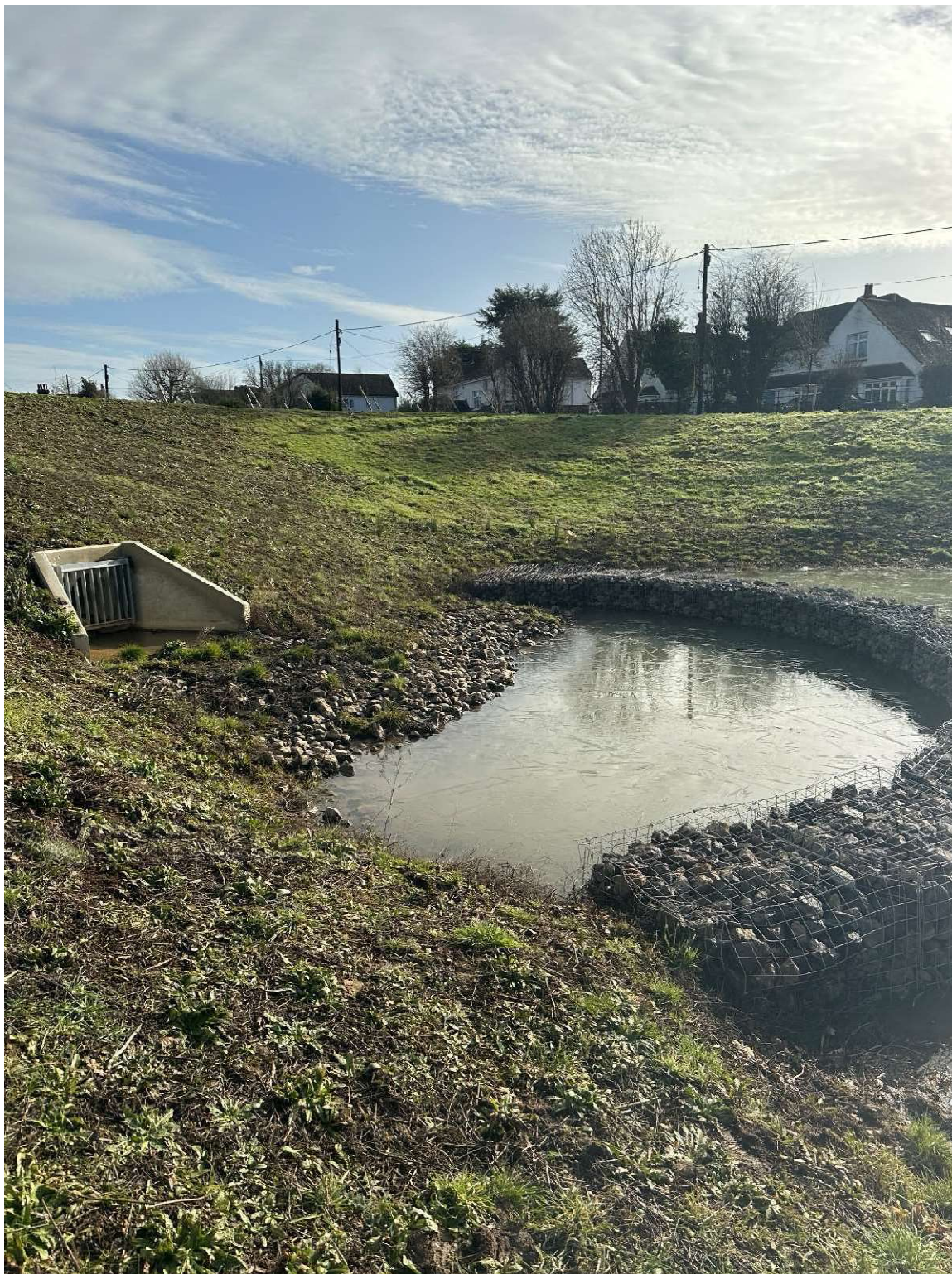
Eastern Pond / Head Wall 1J - 01 February 2023 – stilling area complete and functioning.
