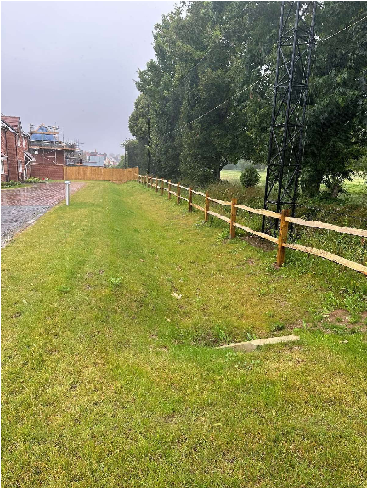
Swale B-HW2A - 9 July 2024 - complete and functioning
