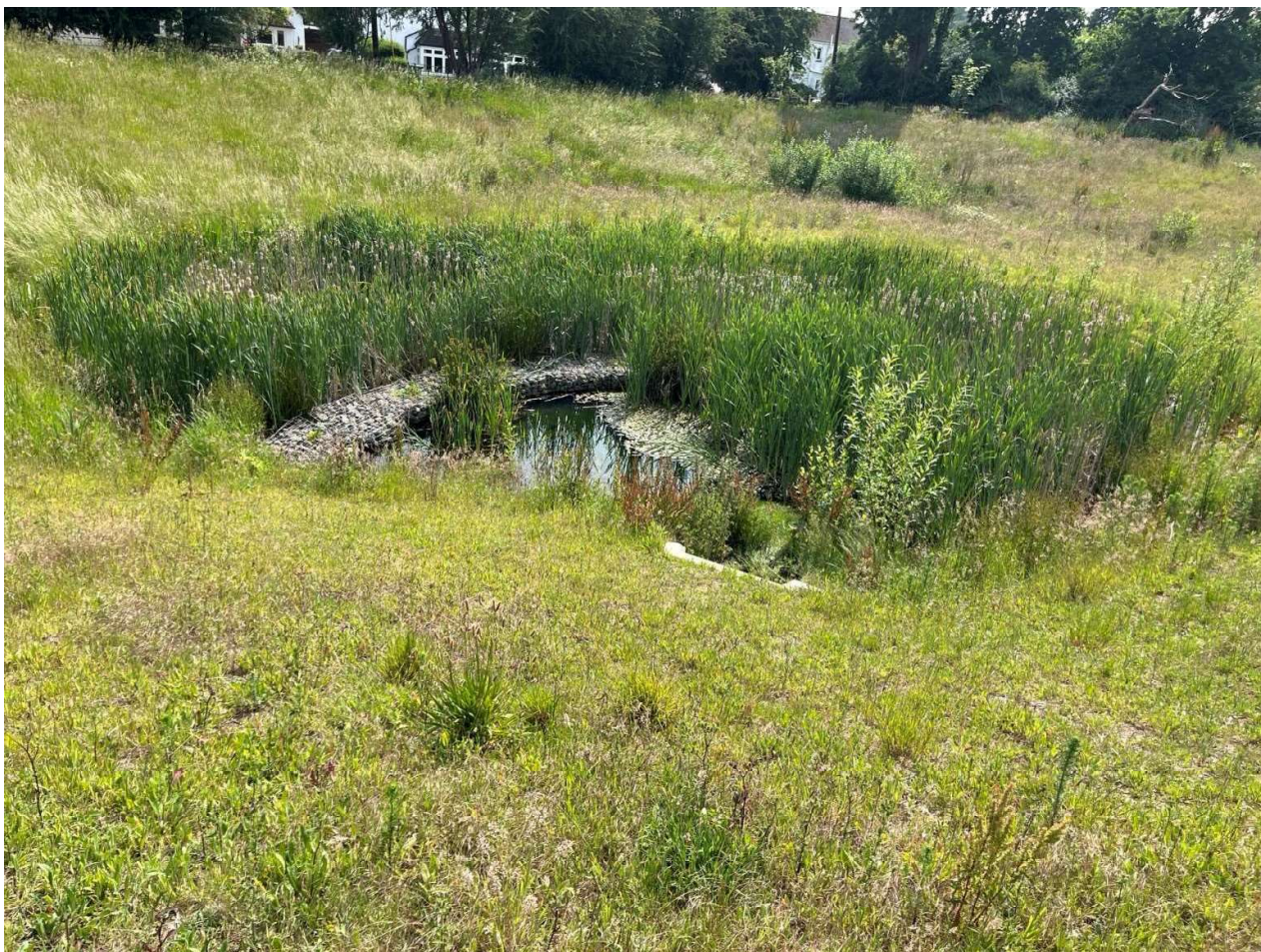
Eastern Pond A - 9 July 2024 - Complete & functioning.
