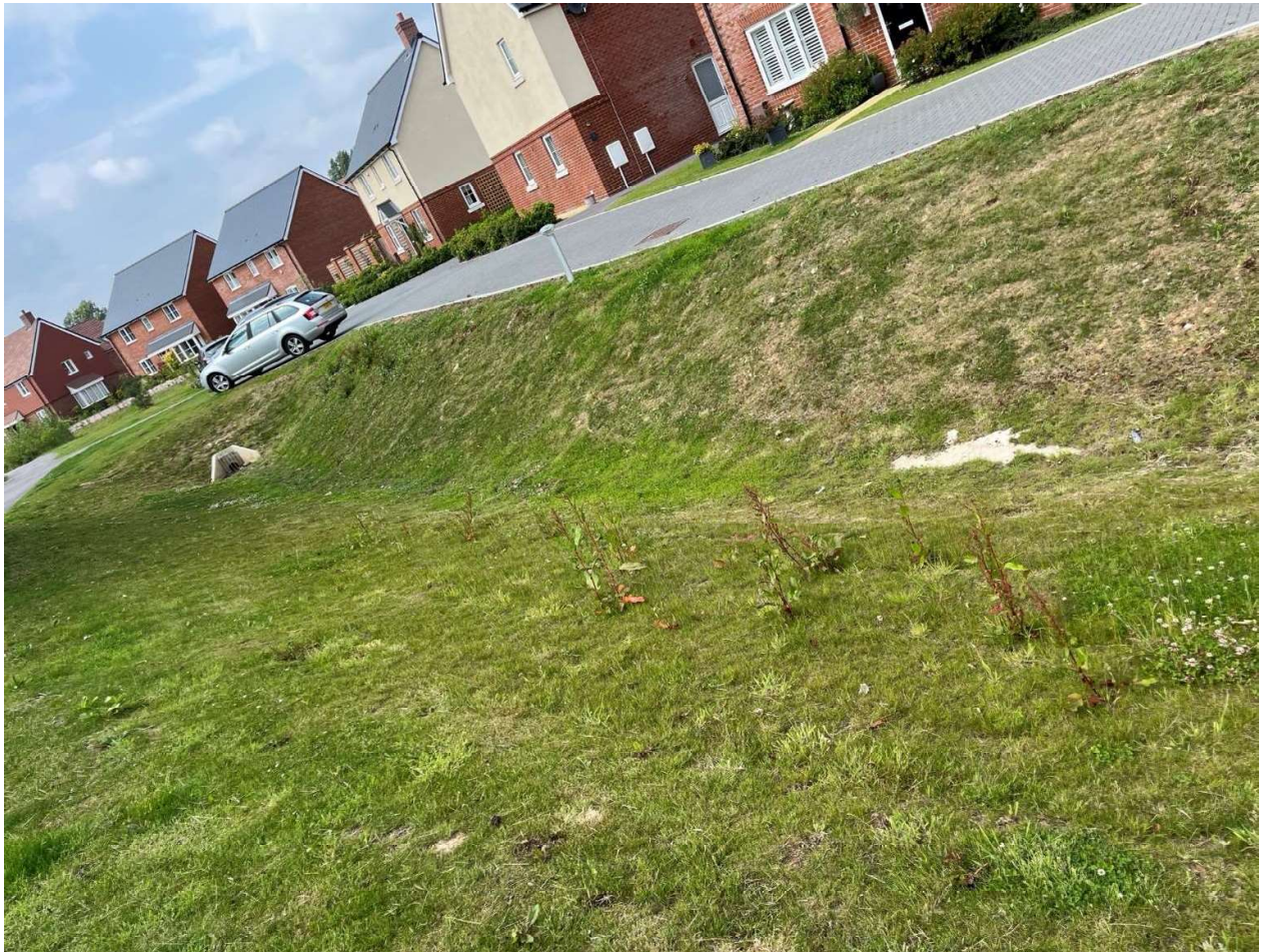
Head Wall 1F - 01 February 2023 – Partially complete. 9 July 2024 - Complete & functioning.
