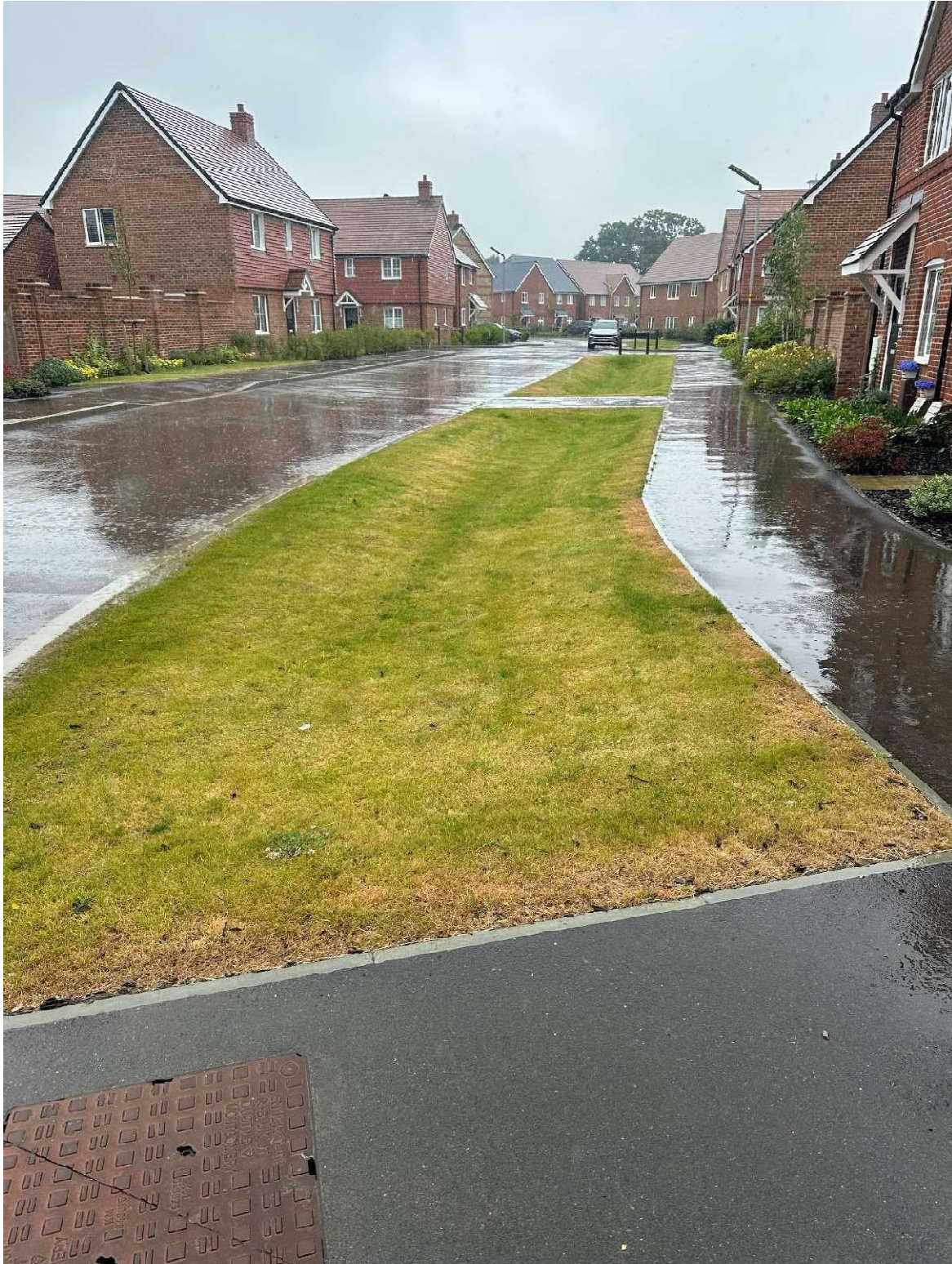
Swale O-N - 9 July 2024 - complete and functioning
