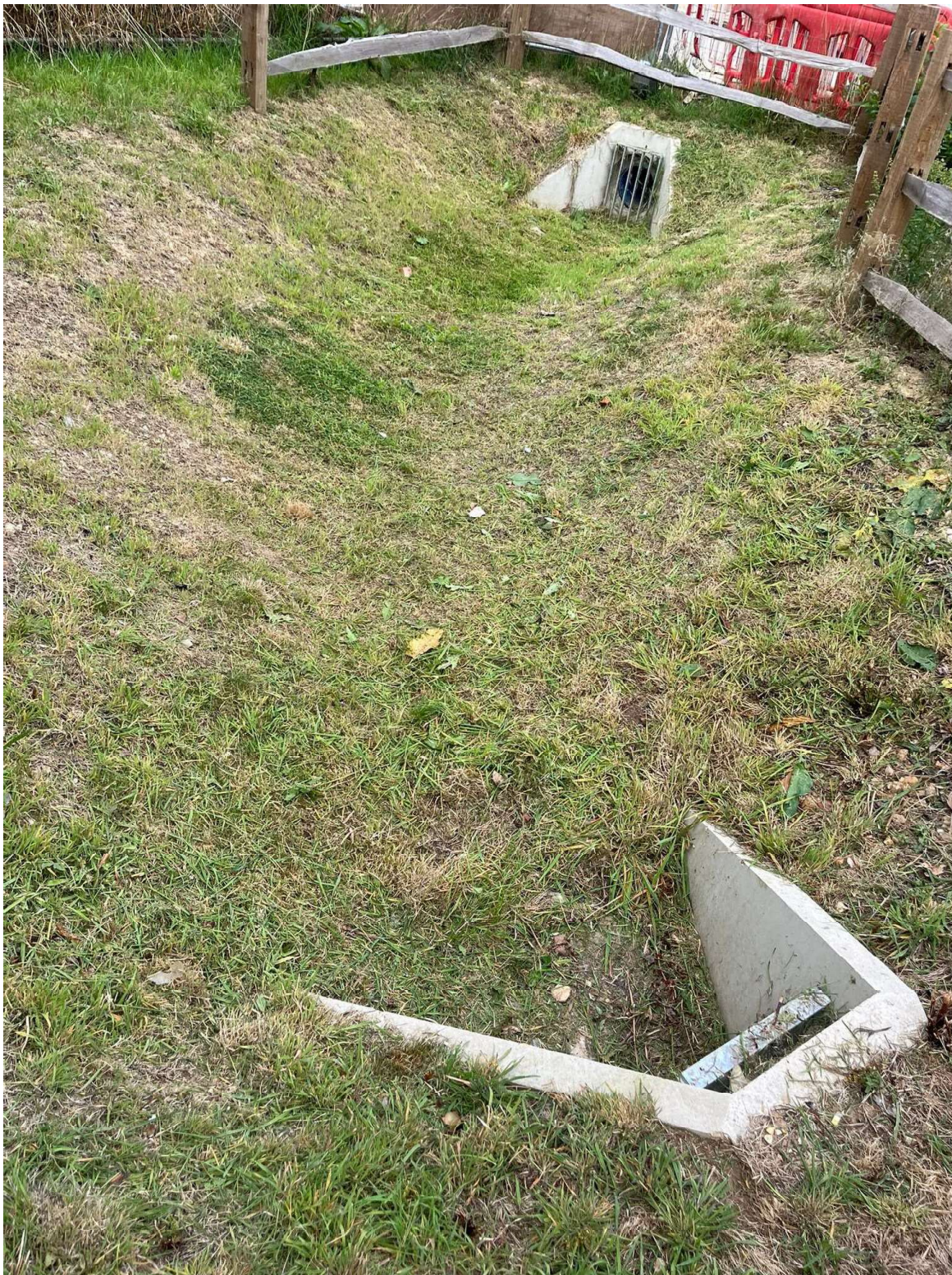
Swale Y – 16 th July 2025 - complete and functioning
