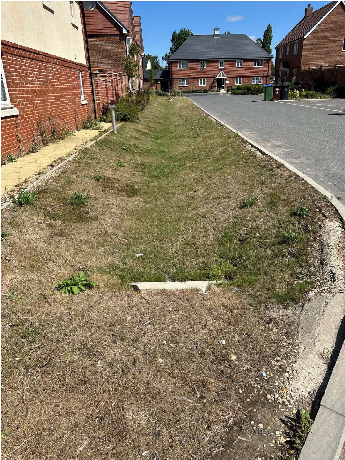
Swale X – 16 th July 2025 - complete and functioning
