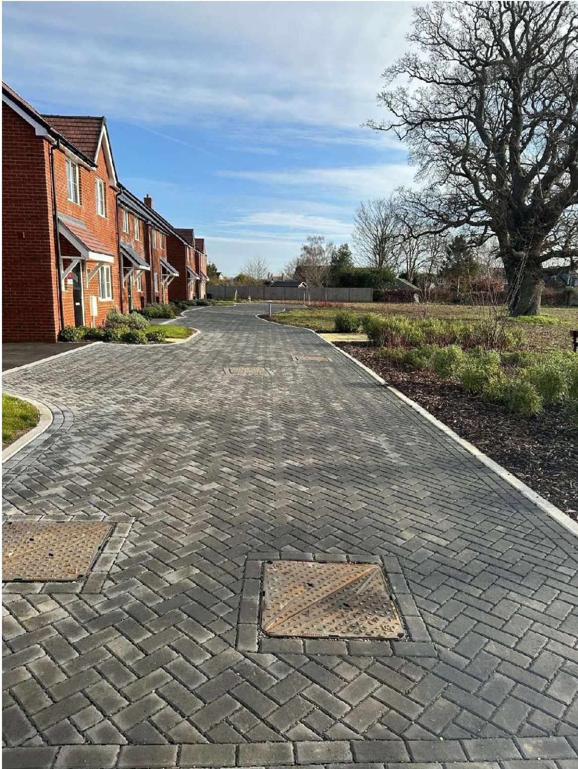
Permeable Paving 1C - 01 February 2023 - complete and functioning
