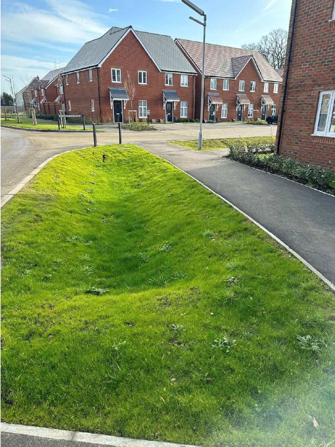
Swale M - - 01 February 2023 - complete and functioning
