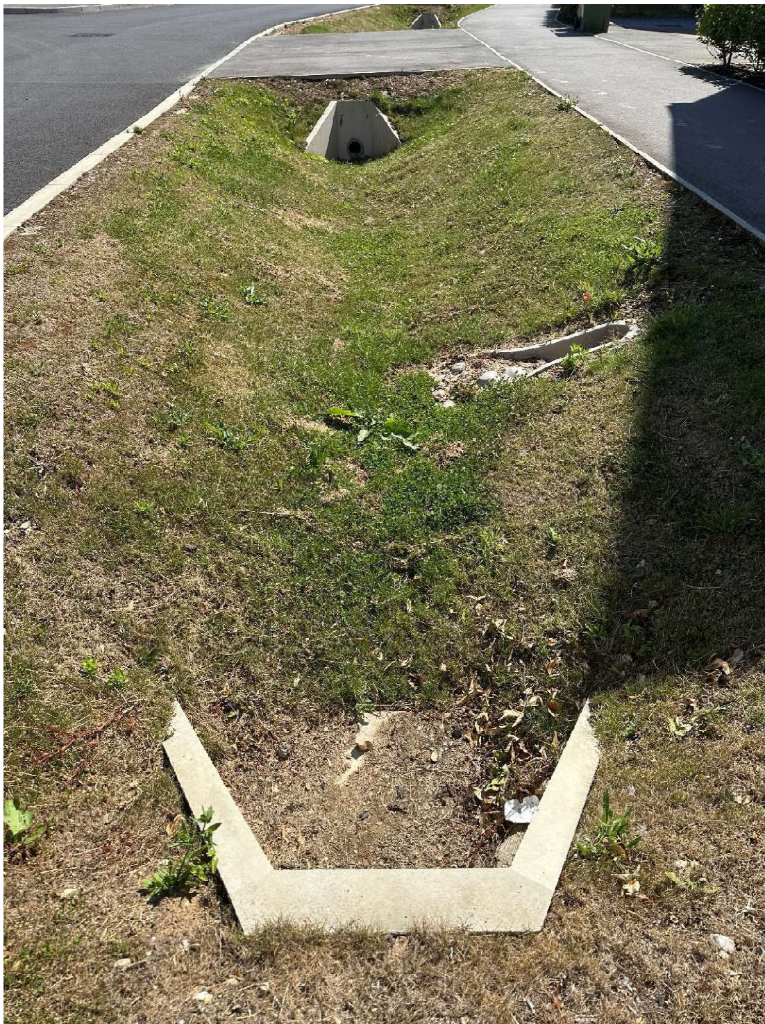
Swale W – 16 th July 2025 - complete and functioning
