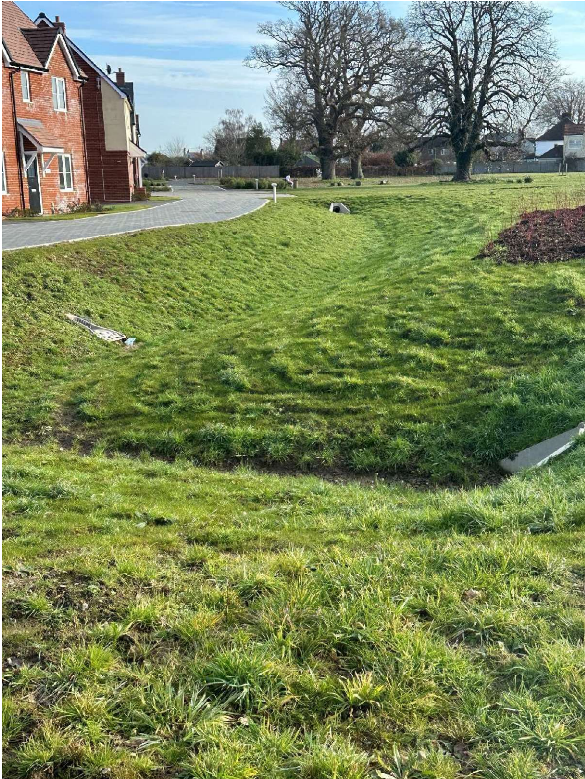
Swale 1H - 01 February 2023 - complete and functioning
