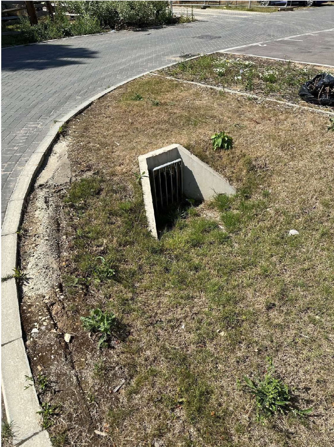
Headwall 3G – 16 th July 2025 - complete and functioning
