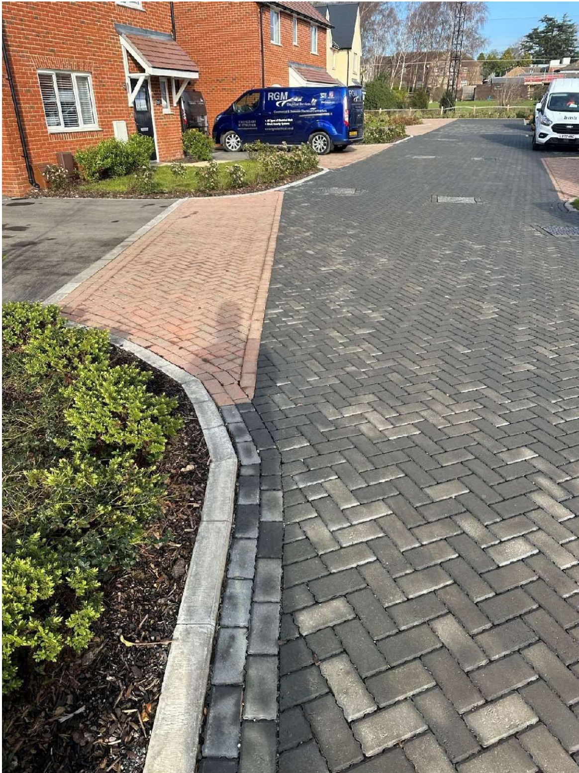
Permeable Paving -1B - 01 February 2023 - complete and functioning
