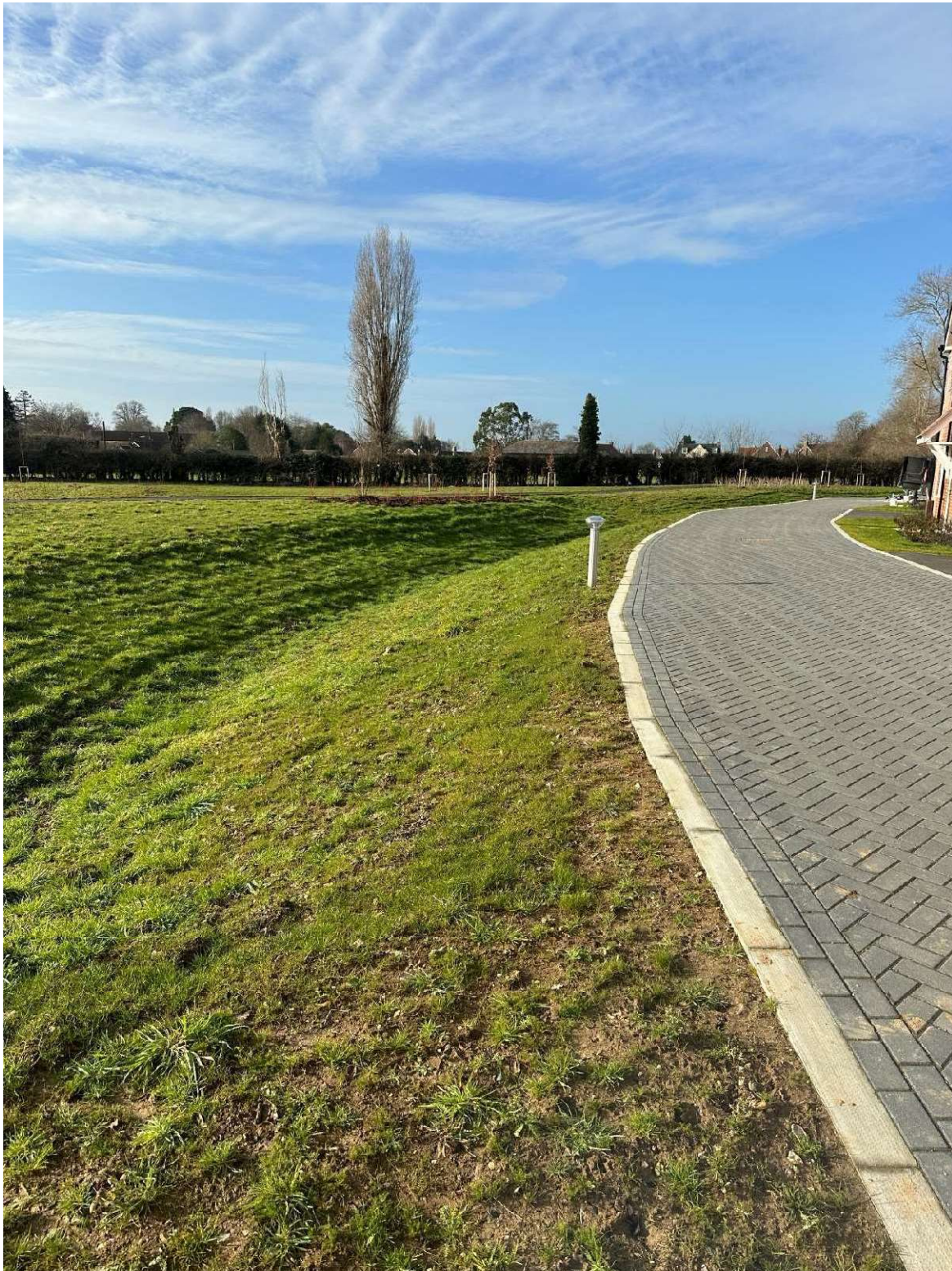
Swale H - 01 February 2023 - complete and functioning
