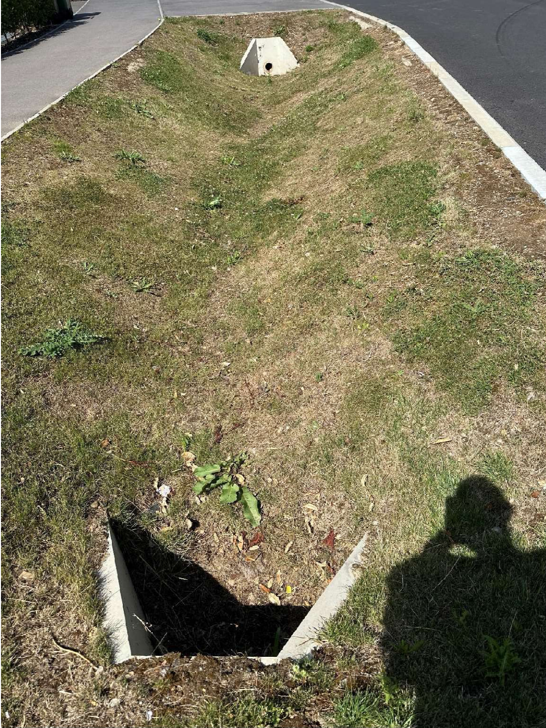
Swale V – 16 th July 2025 - complete and functioning
