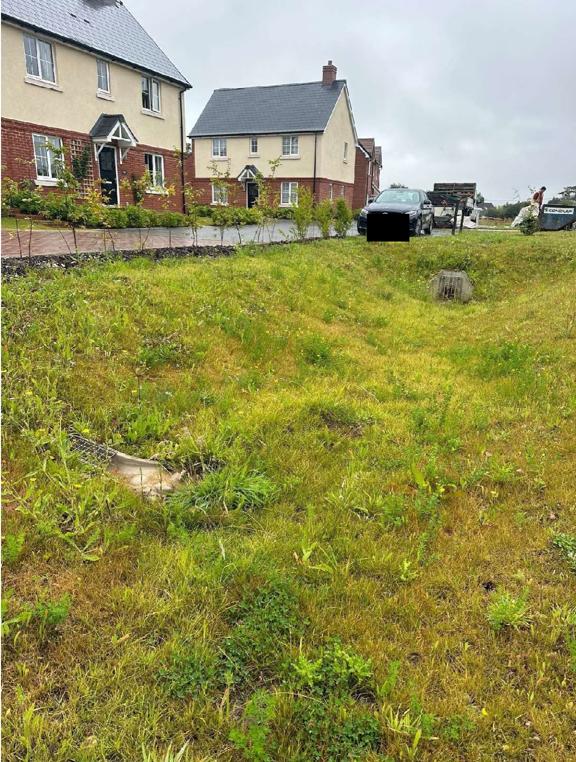
Swale S-HW2F - 9 July 2024 - complete and functioning
