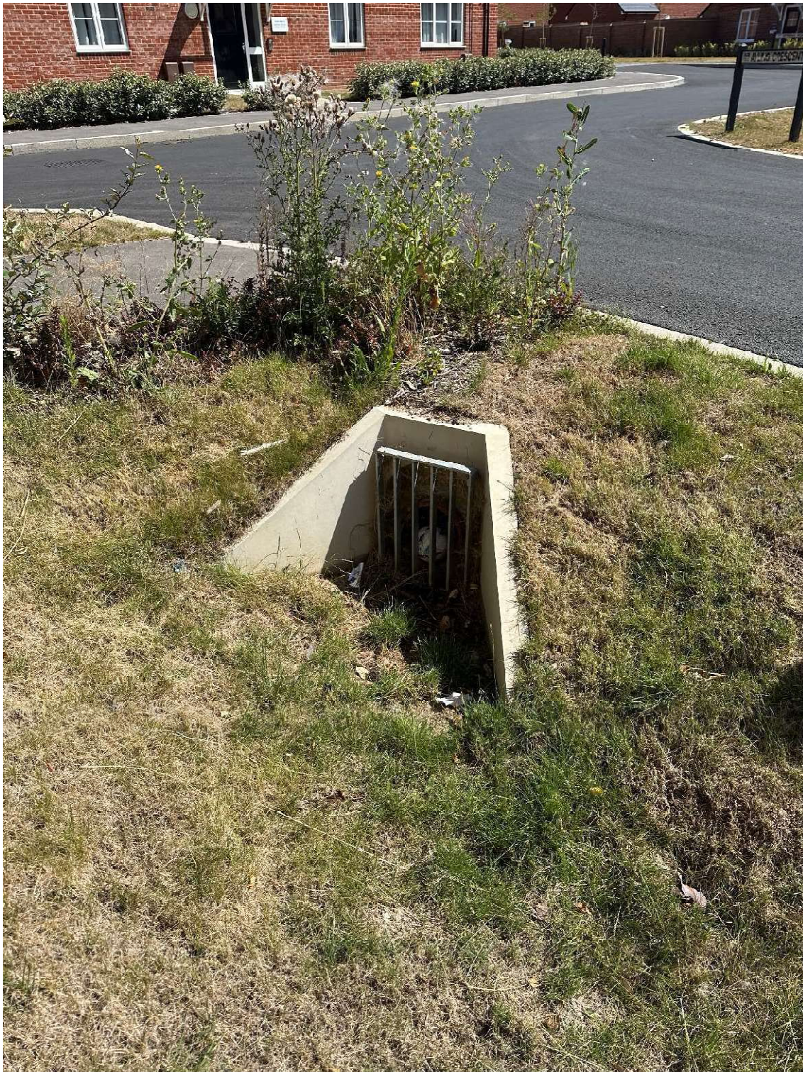
Headwall 3H – 16 th July 2025 - complete and functioning
