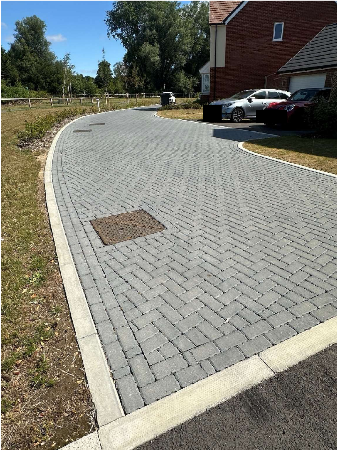
Private parking 4A – 16 th July 2025 - complete and functioning
