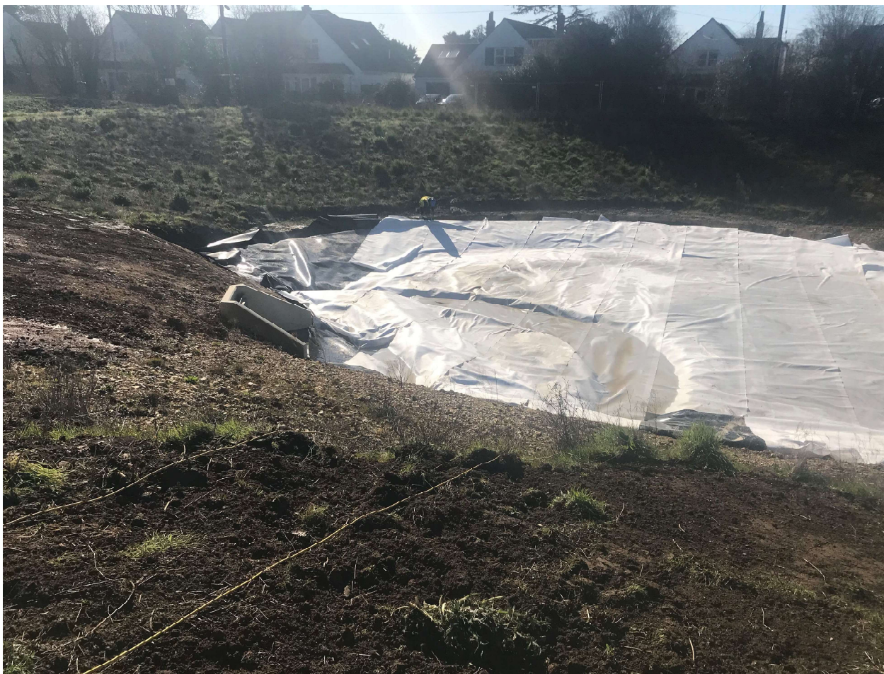
Eastern Pond - 17 March 2022 – under construction, liner being installed.
