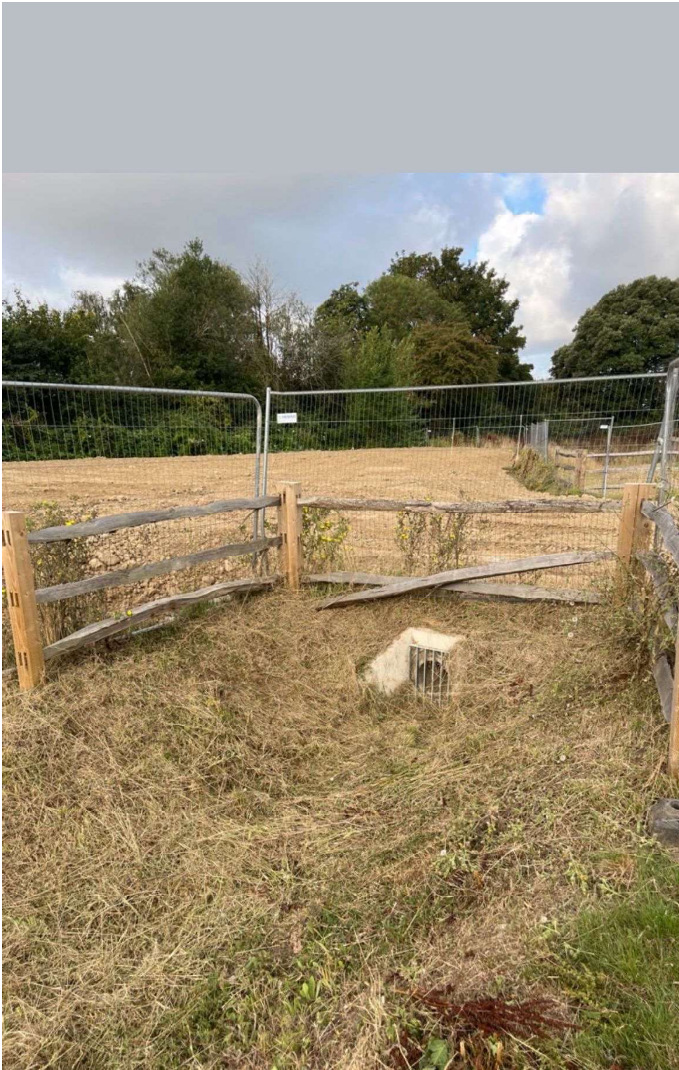
Headwall 3C – 16 th July 2025 - complete and functioning
