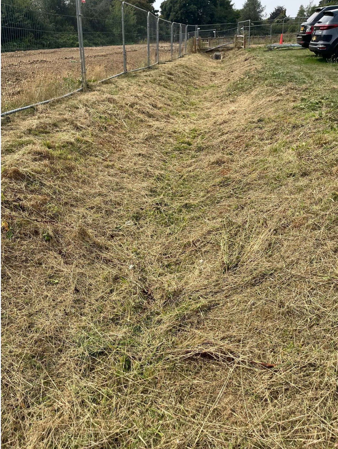
Swale Z – 16 th July 2025 - complete and functioning
