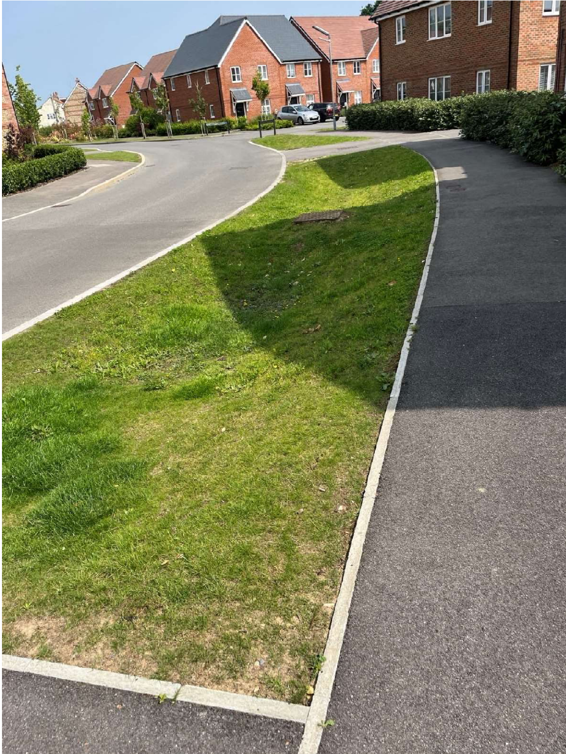
Swale K / L - 01 February 2023 Partially complete. 9 July 2024, complete & functioning.
