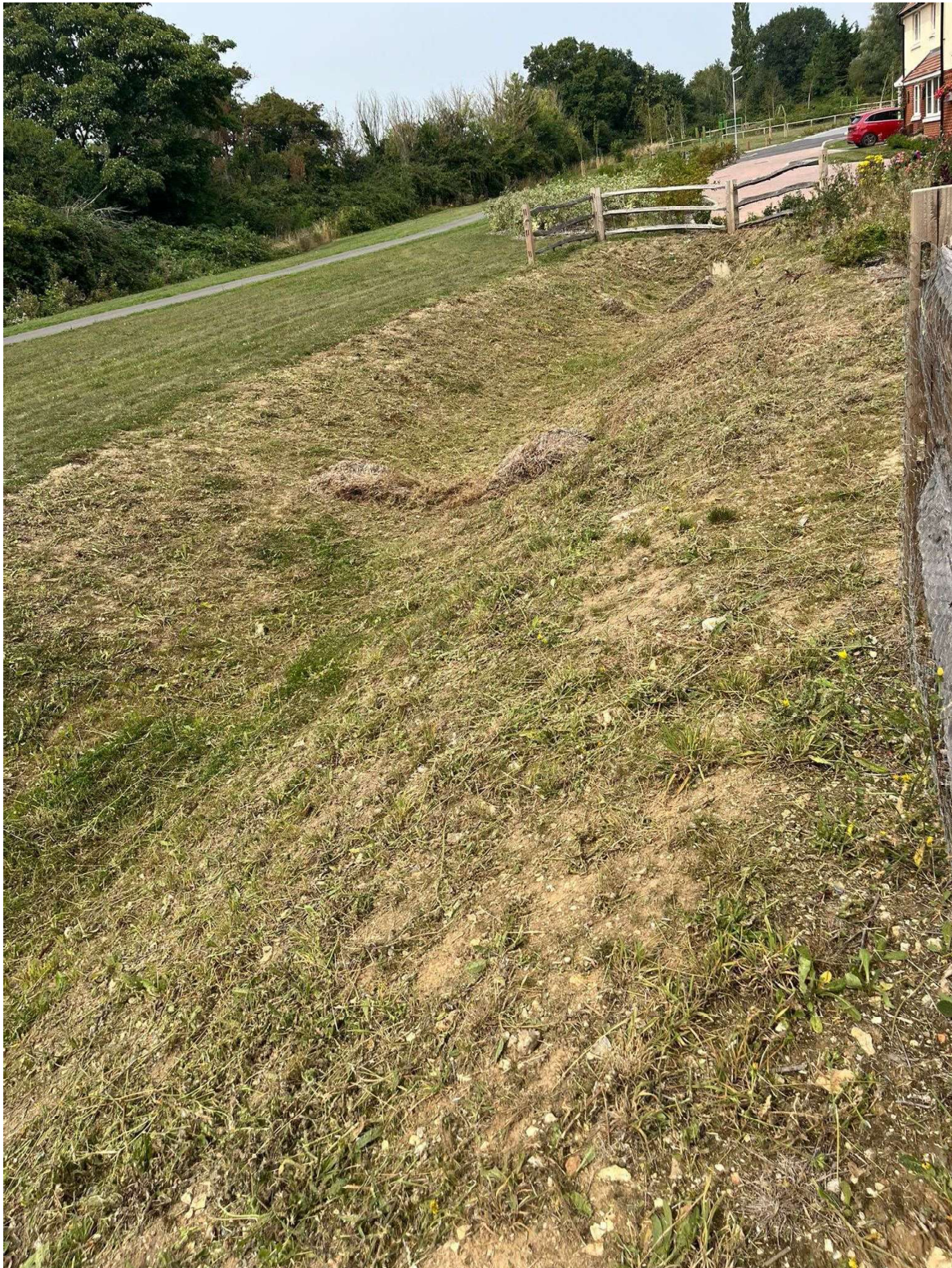
Swale A/B – 16 th July 2025 - complete and functioning
