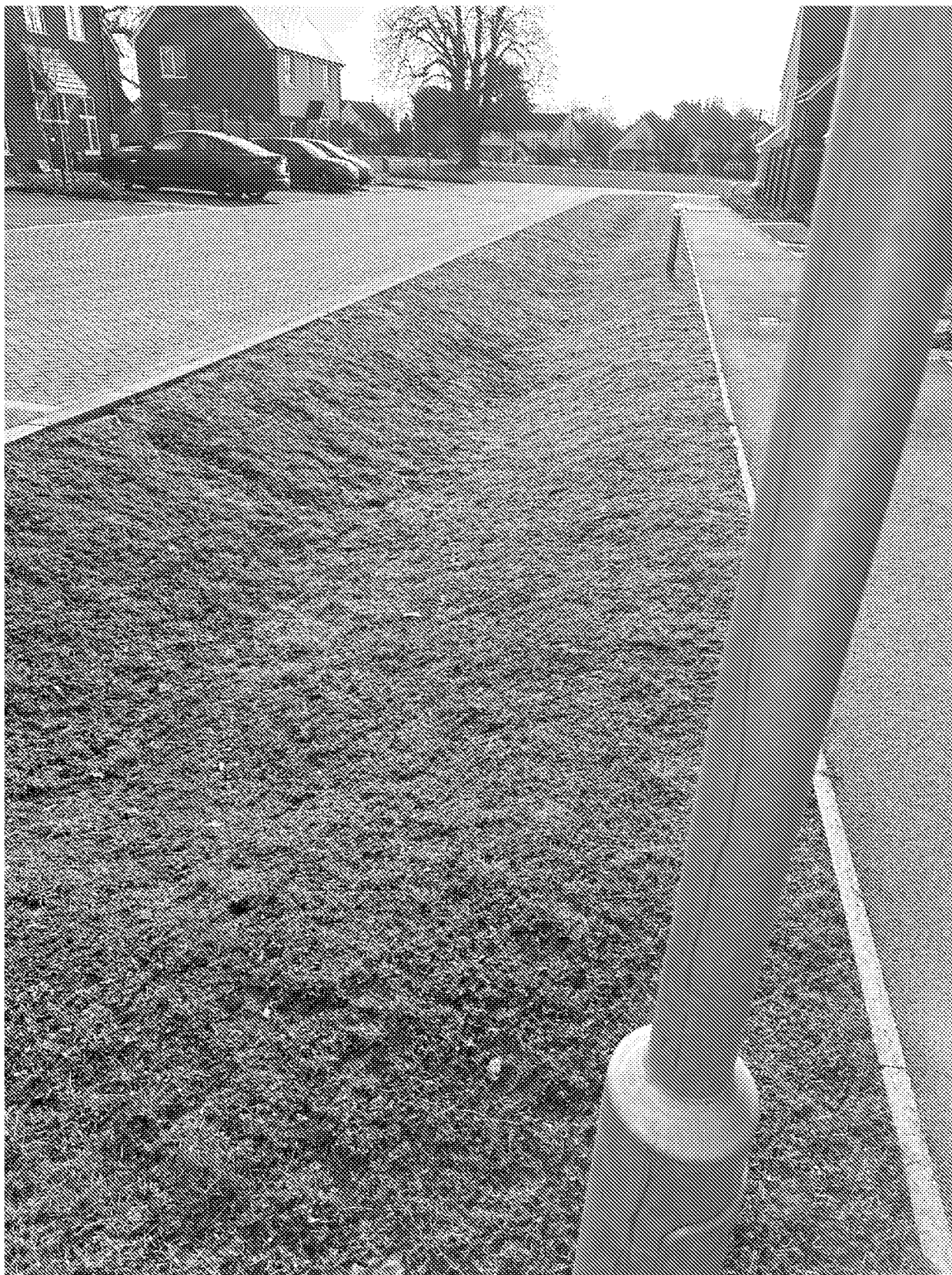
Swale I - 01 February 2023 – complete and functioning
