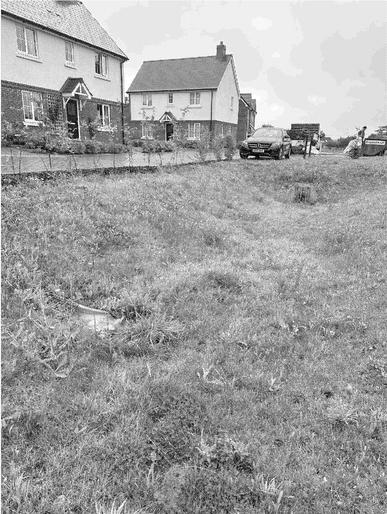
Swale S-HW2F - 9 July 2024 - complete and functioning
