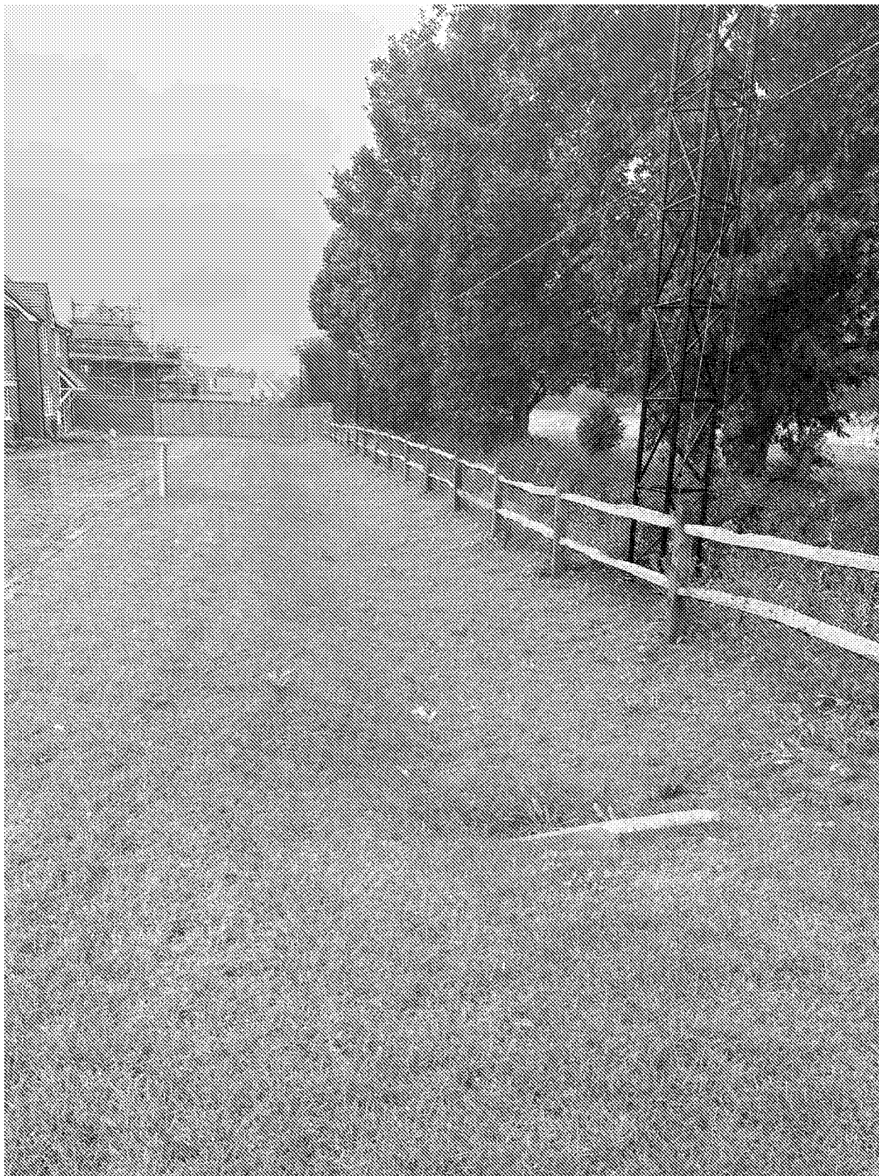
Swale B-HW2A - 9 July 2024 - complete and functioning
