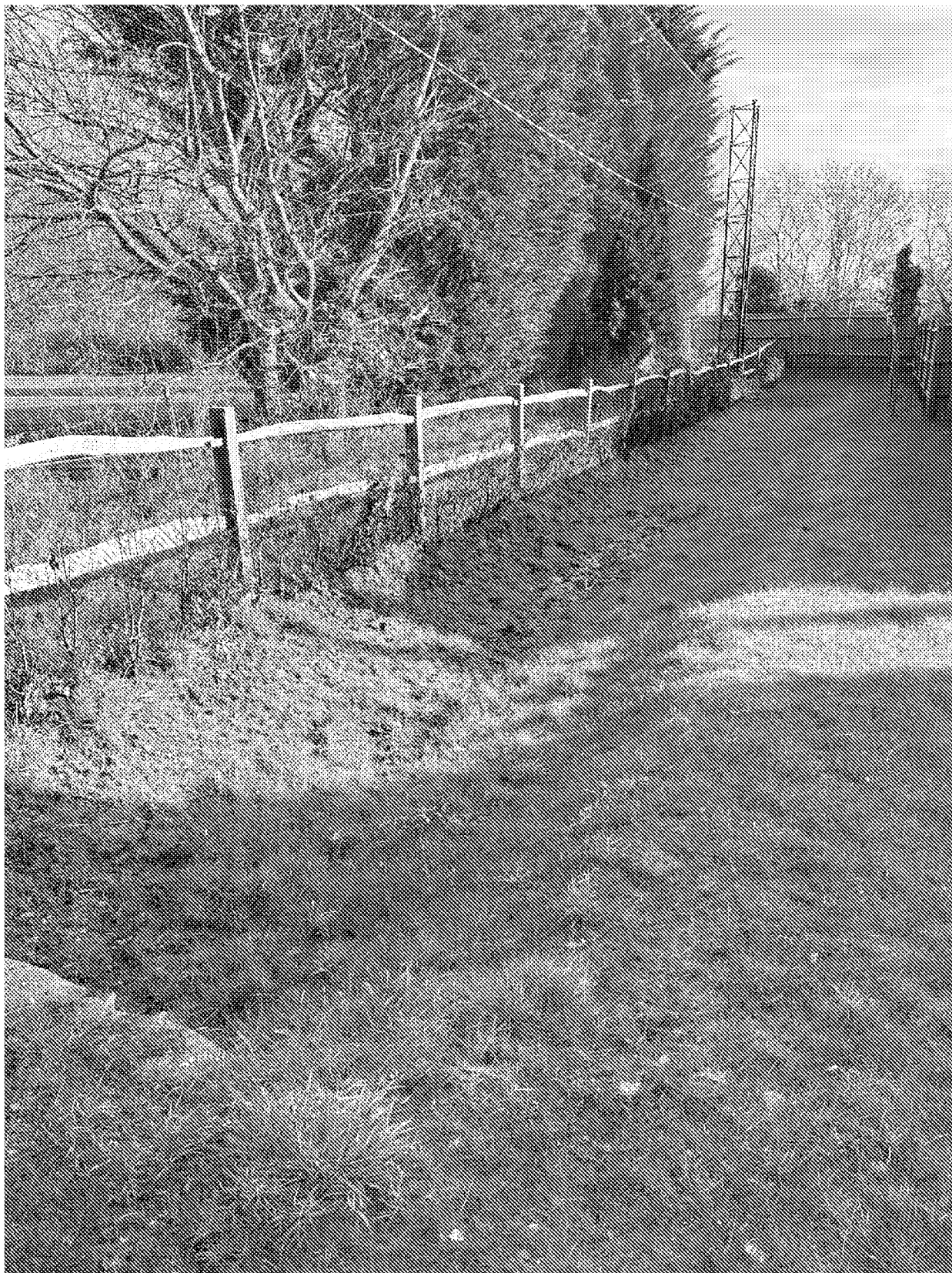
Swale D - 01 February 2023 - complete and functioning
