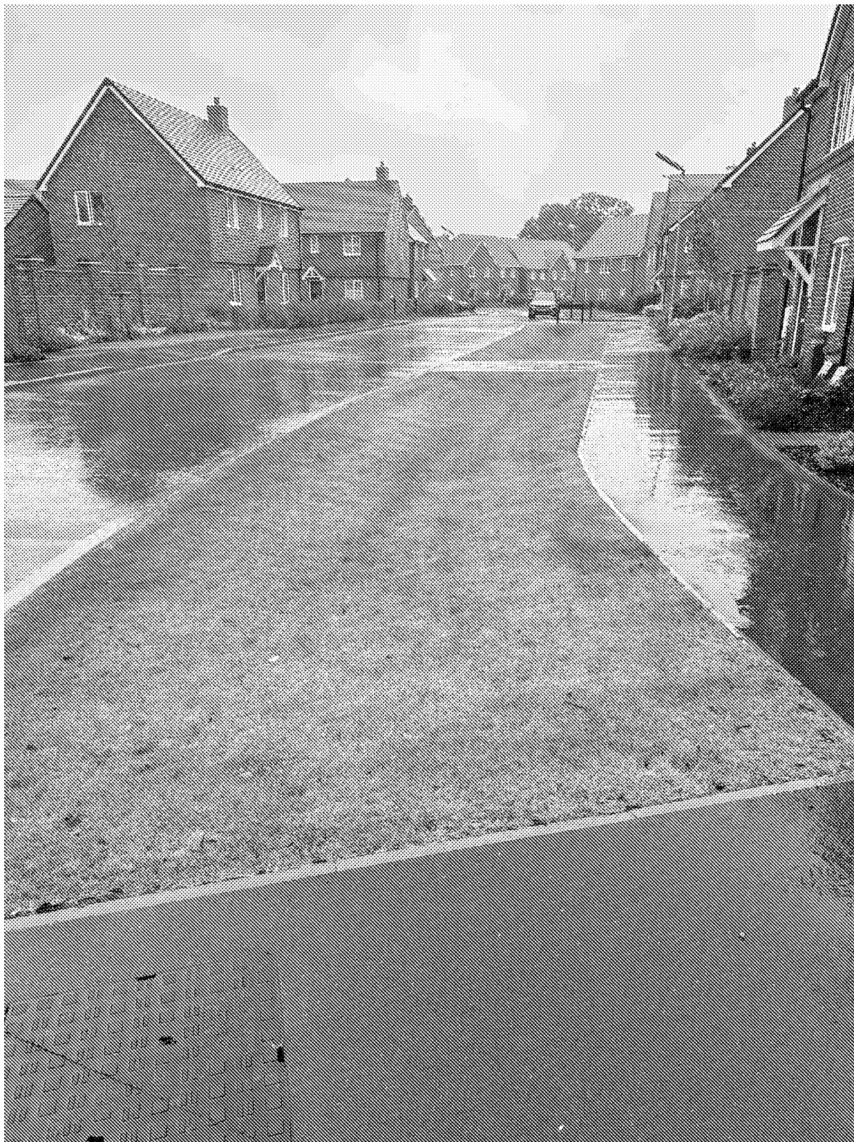
Swale O-N - 9 July 2024 - complete and functioning
