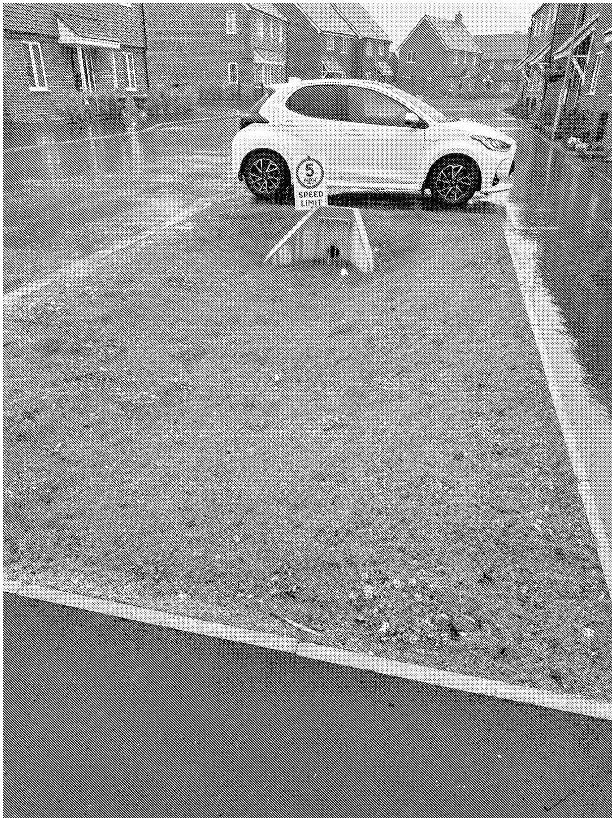
Swale R-HW2G - 9 July 2024 - complete and functioning
