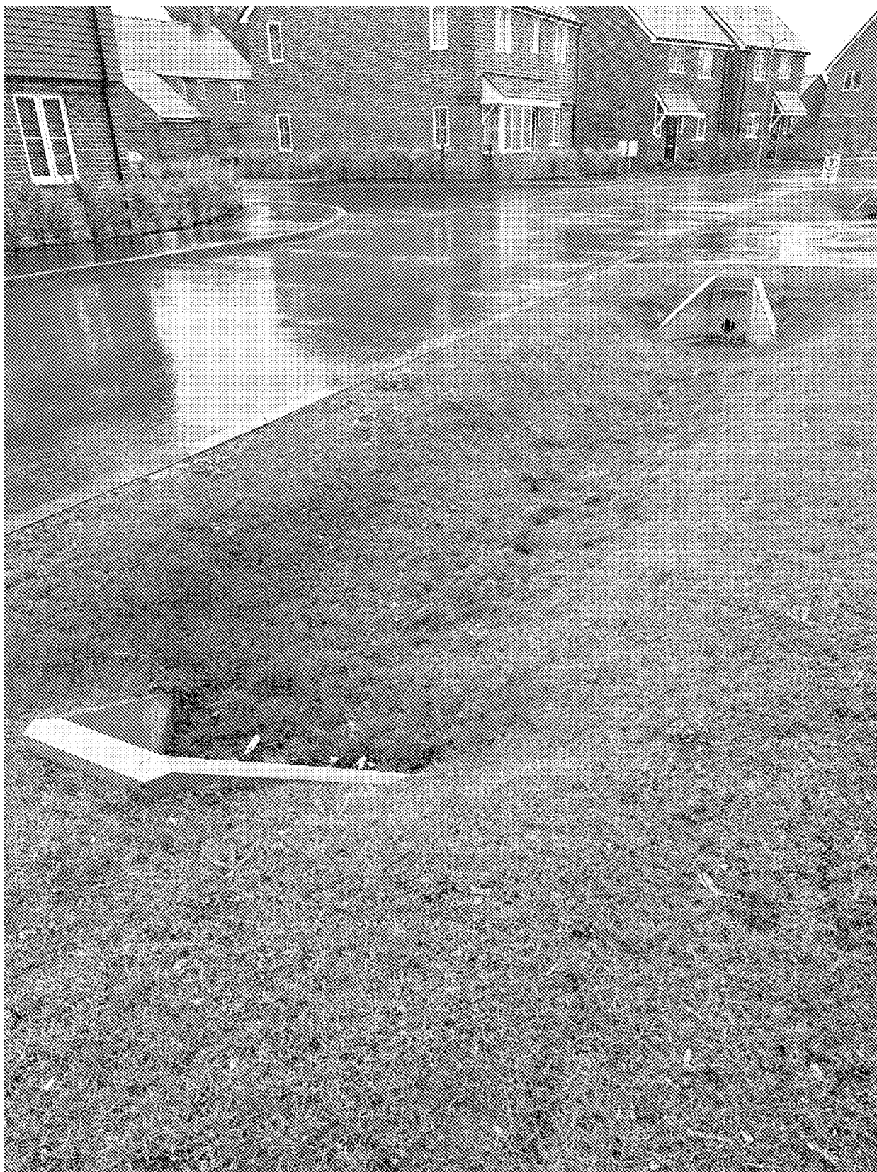
Swale P-Q-HW2C-G - 9 July 2024 - complete and functioning
