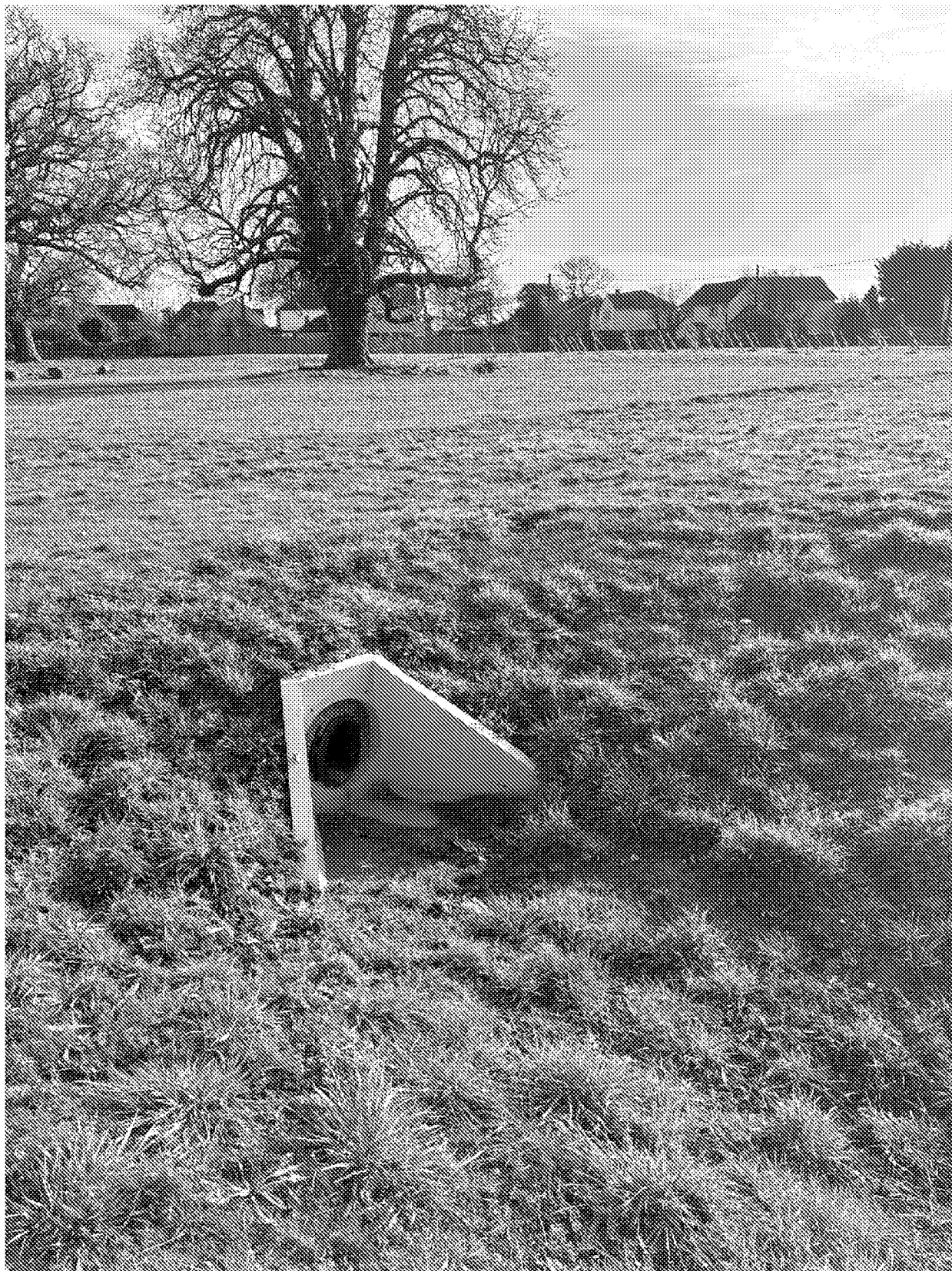
Head Wall 1G - 01 February 2023 - complete and functioning
