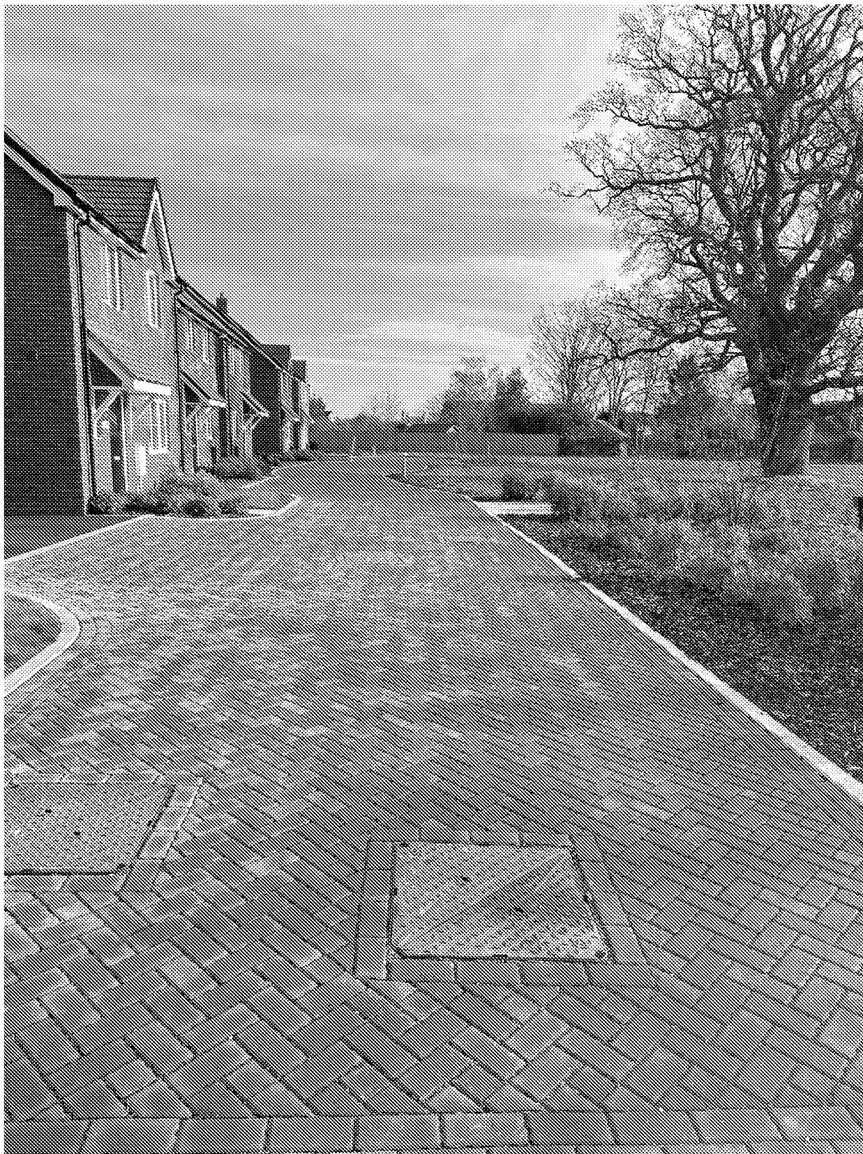
Permeable Paving 1C - 01 February 2023 - complete and functioning
