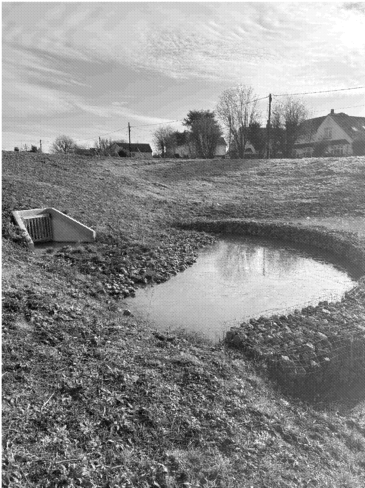
Eastern Pond / Head Wall 1J - 01 February 2023 – stilling area complete an functioning.
