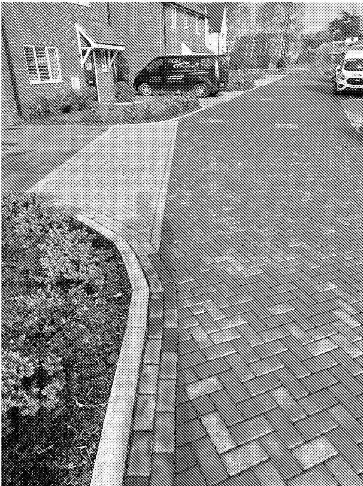
Permeable Paving -1B - 01 February 2023 - complete and functioning
