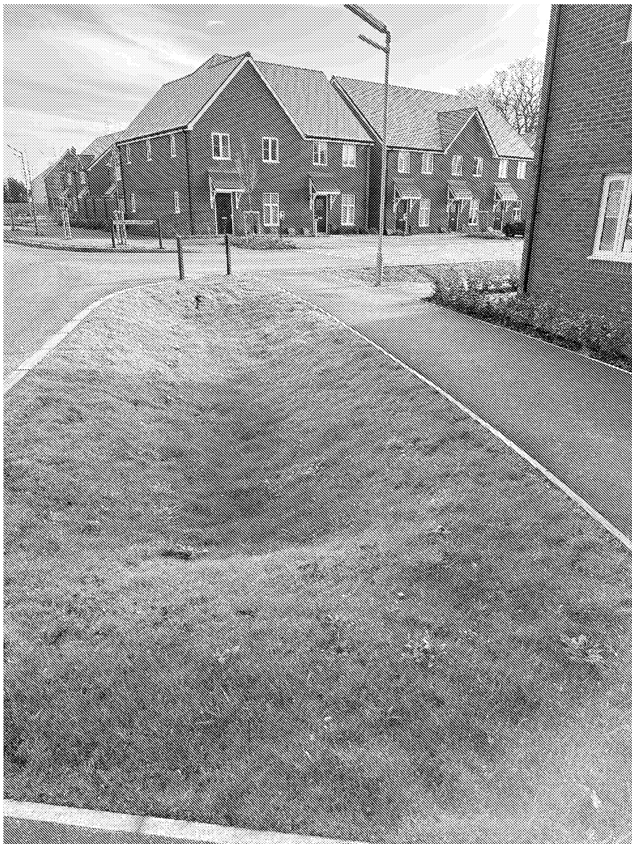
Swale M - - 01 February 2023 - complete and functioning
