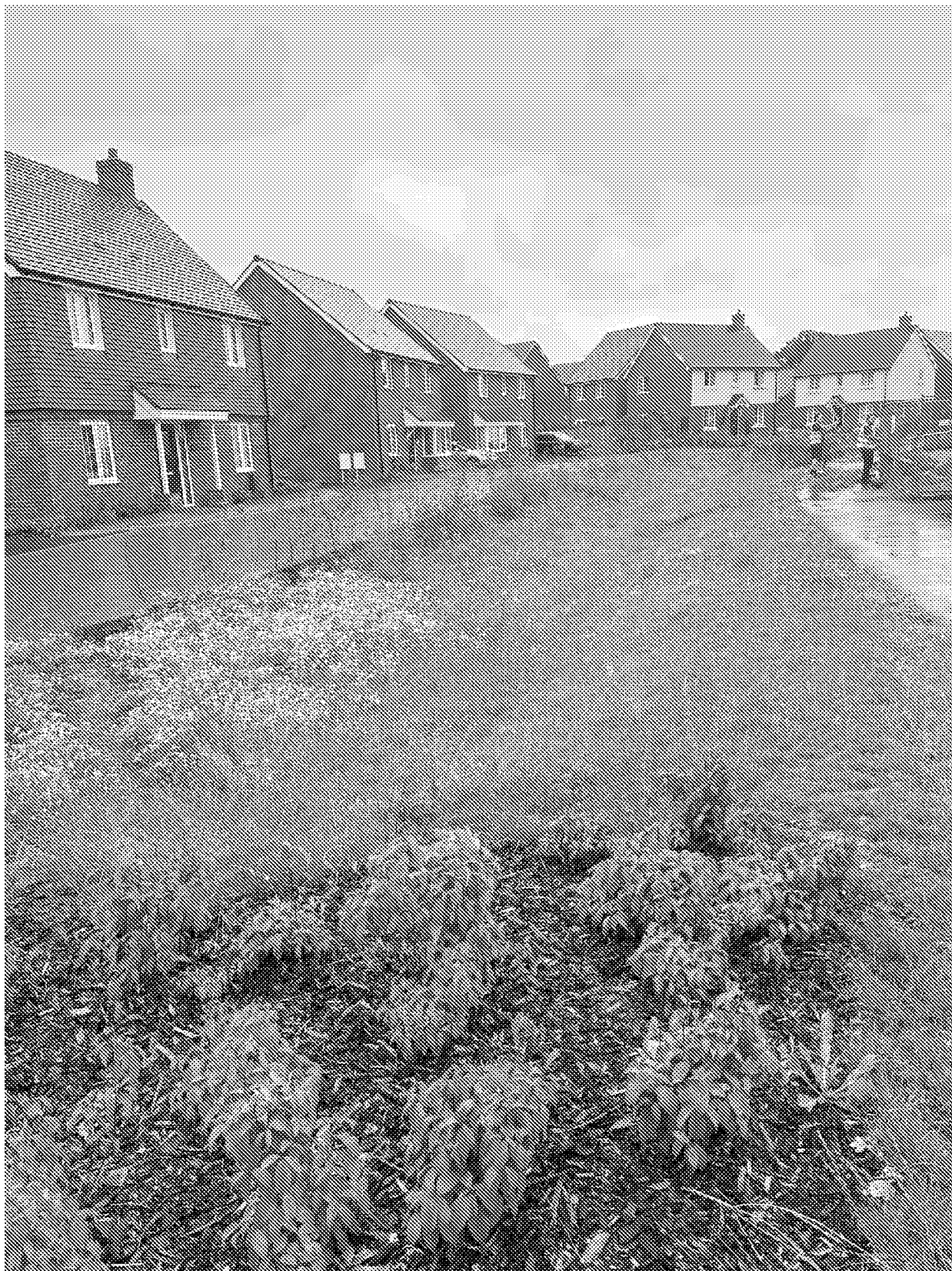
Swale S – 09 July 2024 - complete and functioning
