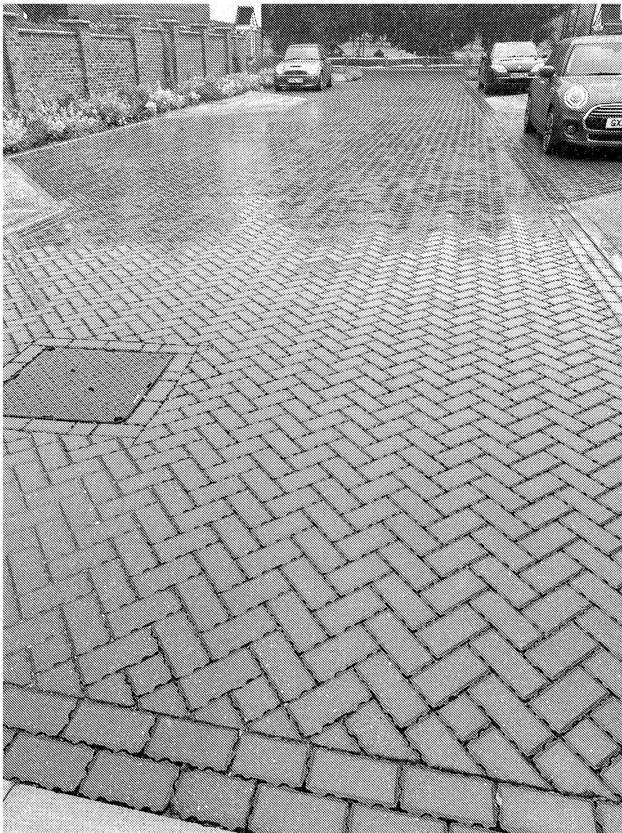
Permeable Pavement 2A - 9 July 2024 - complete and functioning
