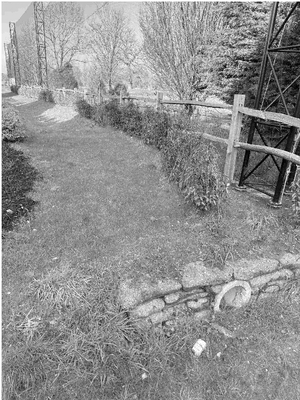
Head Wall 1B - 01 February 2023 - complete and functioning
