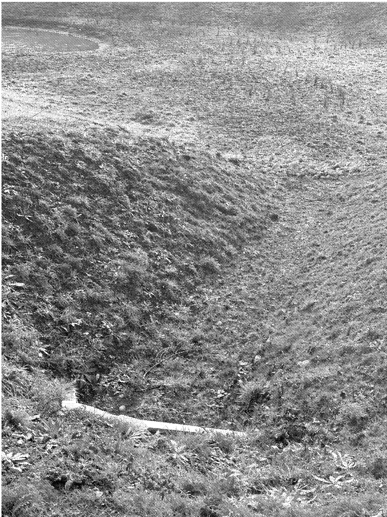
Swale G and Head Wall 11 - 01 February 2023 - complete and functioning
