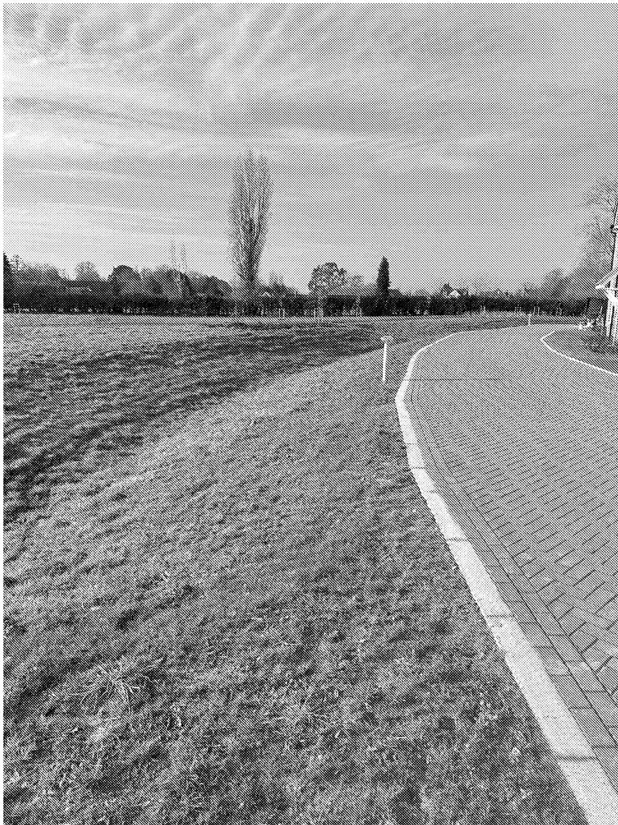
Swale H - 01 February 2023 - complete and functioning
