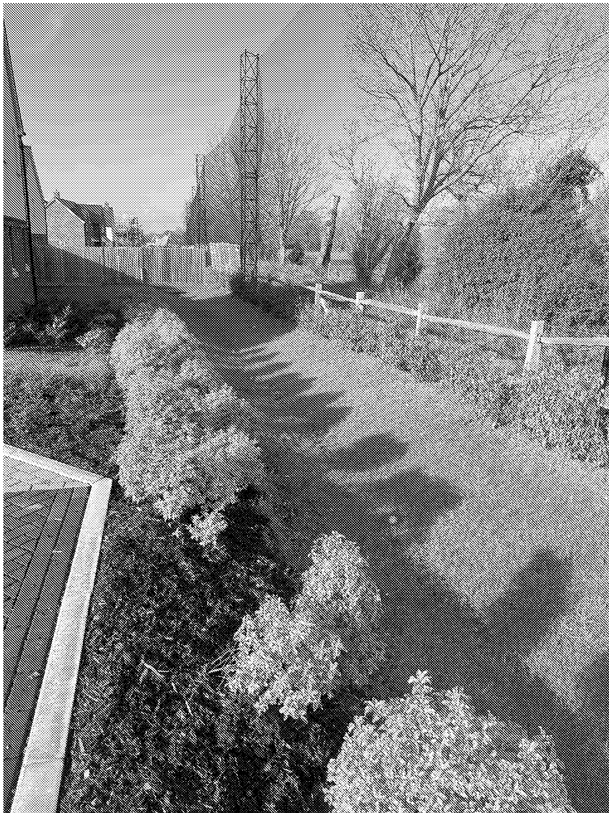
Swale C - 01 February 2023 - complete and functioning
