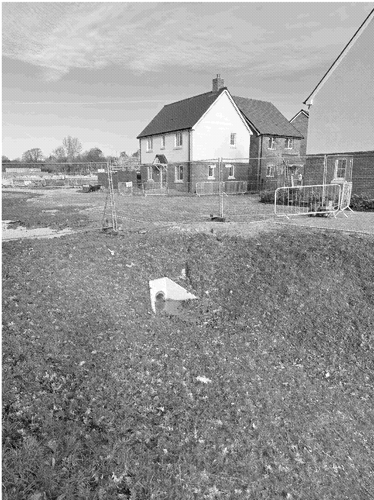
Head Wall 1F - 01 February 2023 – Partially complete
