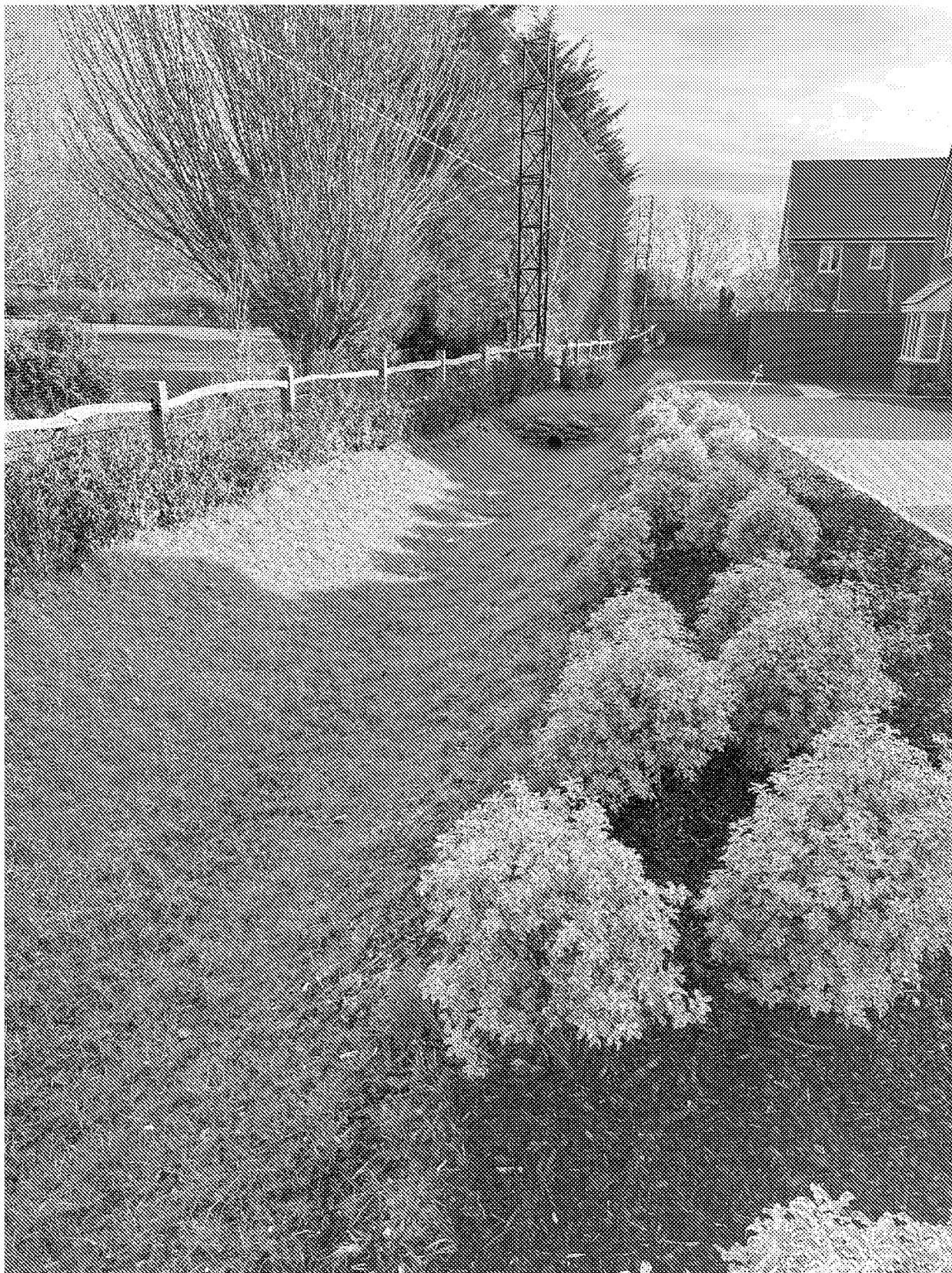
Swale C and Head Wall 1A - 01 February 2023 - complete and functioning
