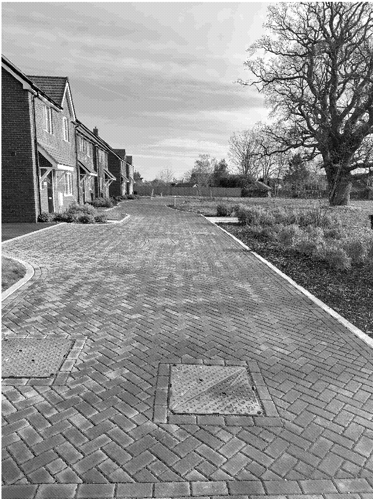
Permeable Paving 1C - 01 February 2023
