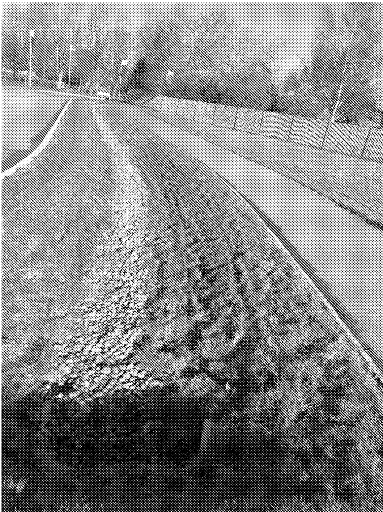
Swale E - 17 January 2022
