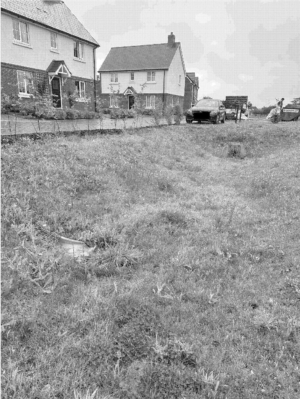
Swale S-HW2F - 9 July 2024
