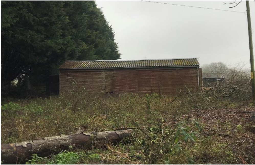
Plate X : Timber outbuilding – West elevation
