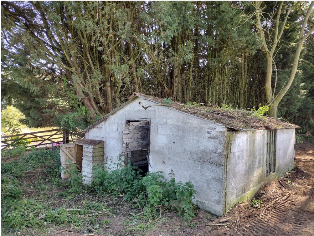
Plate VIII : Blockwork outbuilding on north boundary - East elevation
