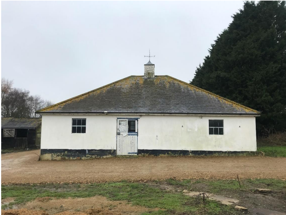
Plate II : Stable Block – East elevation viewed from proposed sand school
