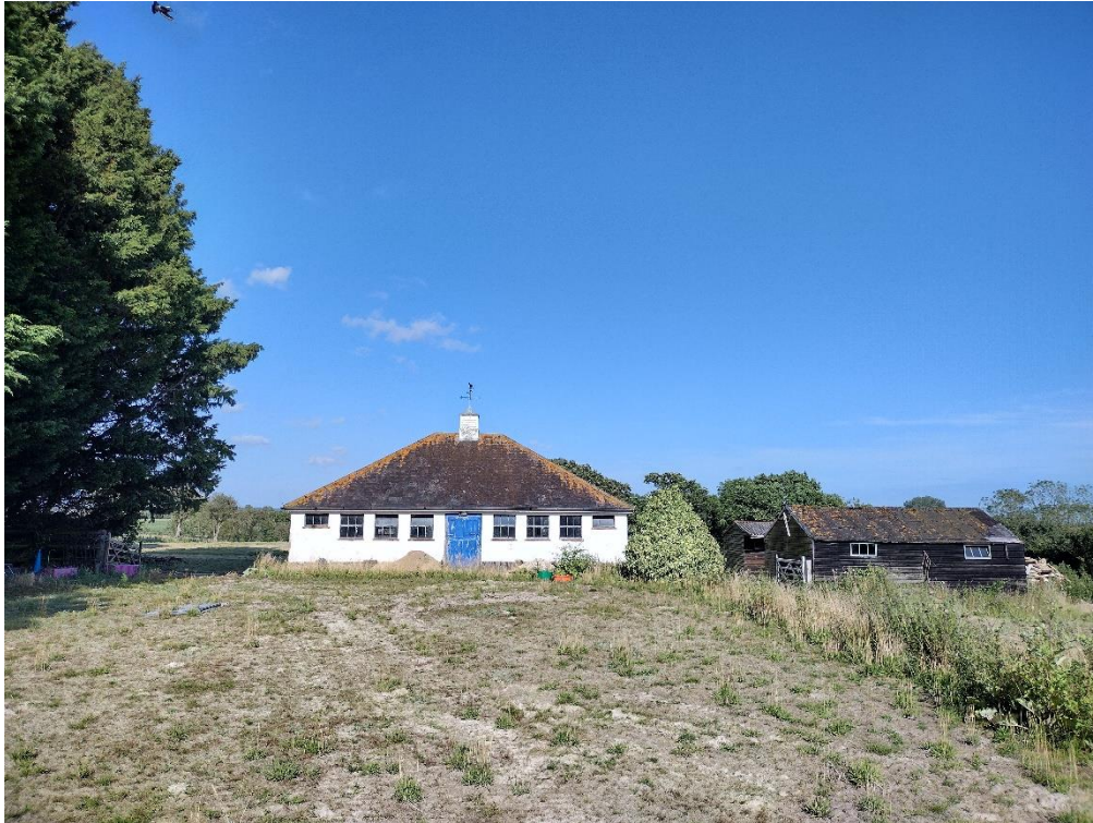
Plate IV : Stable Block – West elevation, with timber stable buildings visible on the right
