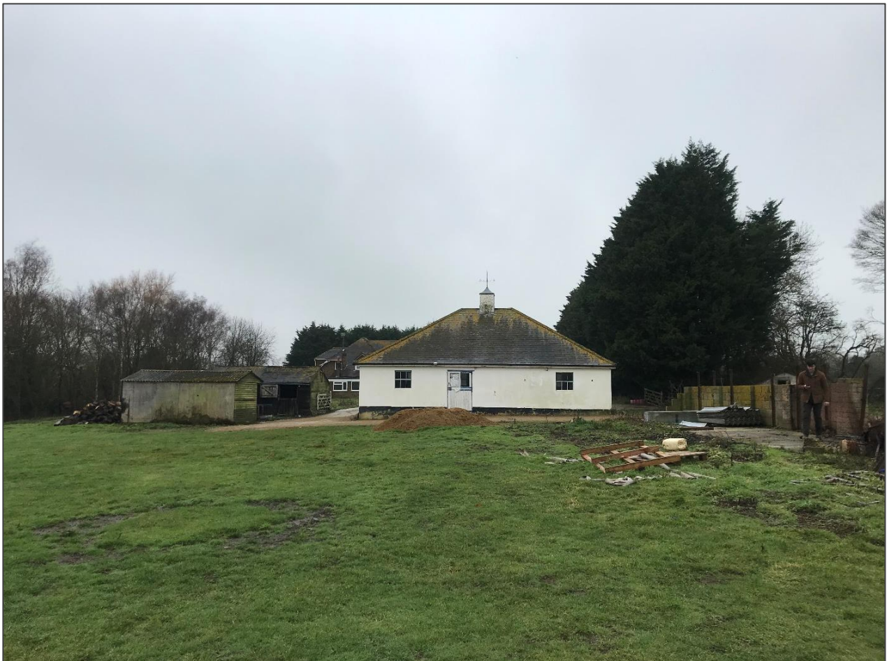
Plate 1 : Stable Block – East elevation viewed from proposed sand school. Timber stables buildings visible on the left.
