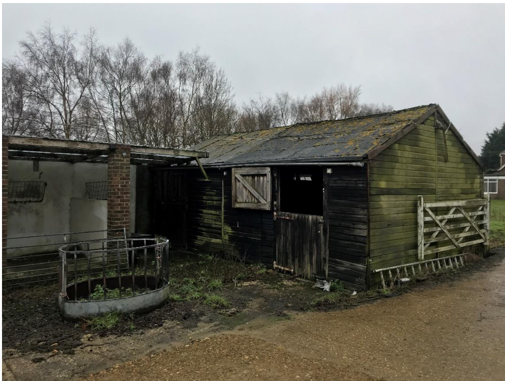
Plate VII : Timber stable buildings – North-east perspective
