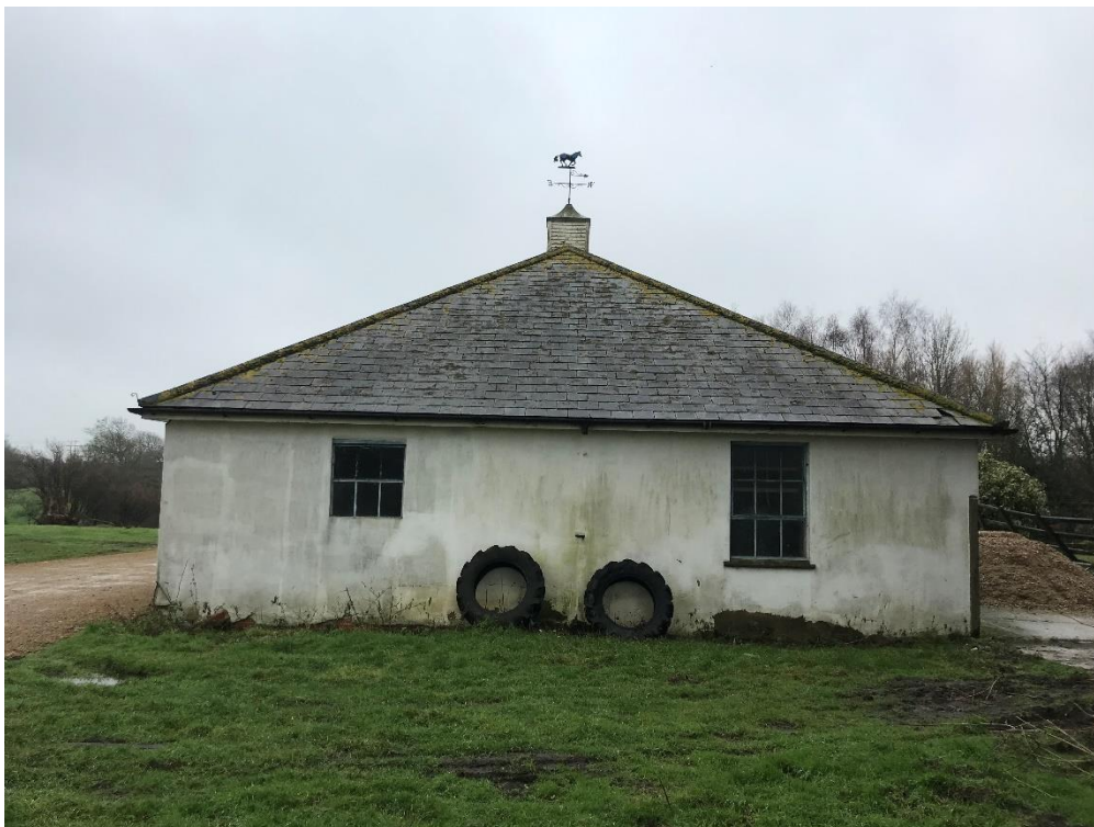
Plate III : Stable Block – North elevation
