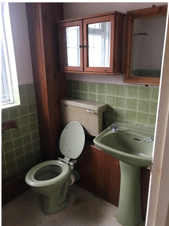
Plate XVII : First floor - bathroom
