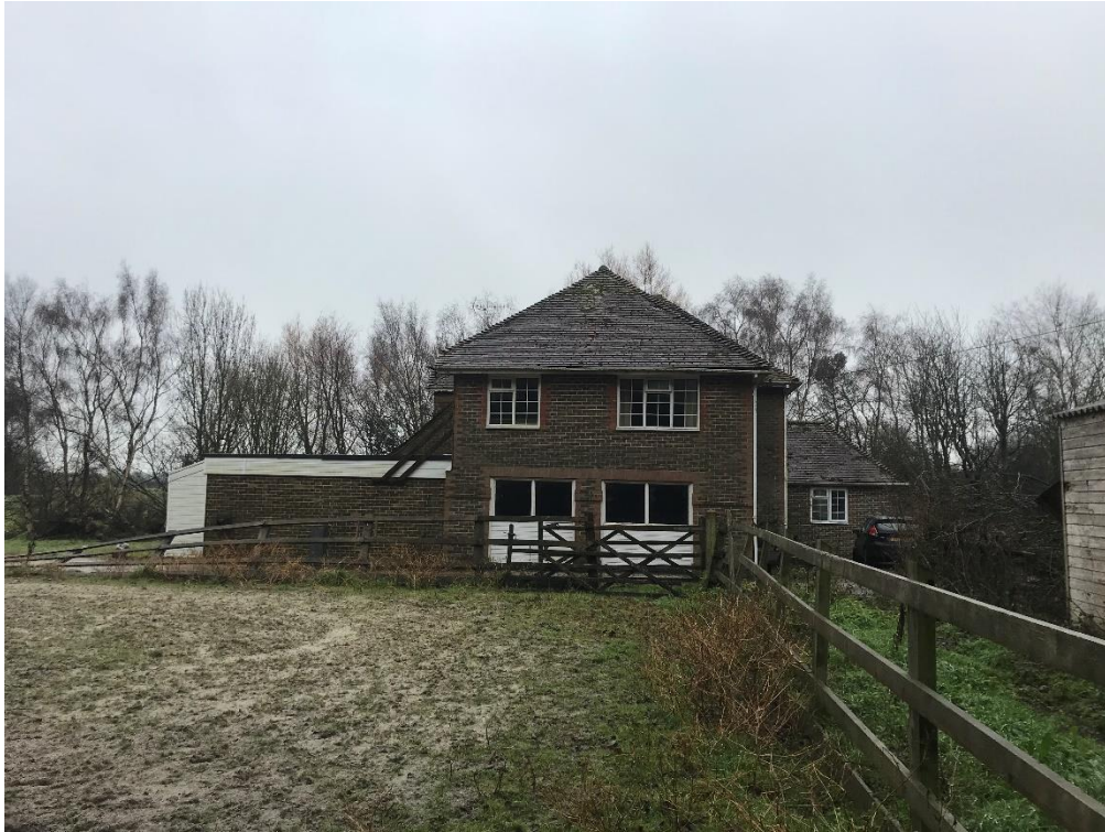
Plate IV : North elevation of existing house
