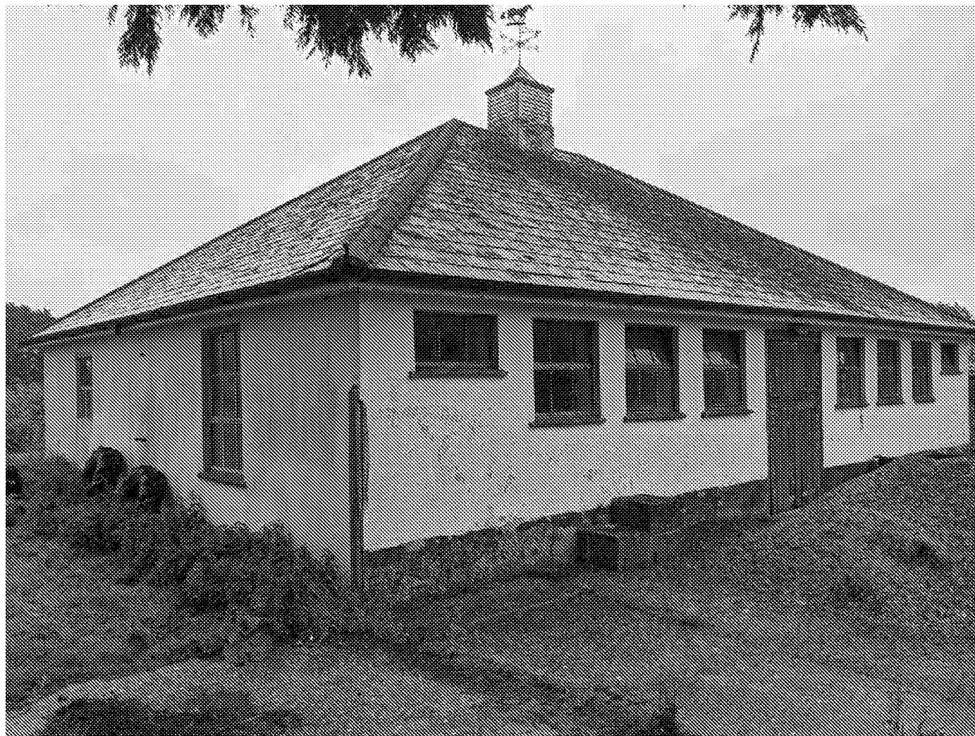
Photo 6 - The building B2, viewed from the north-west.
