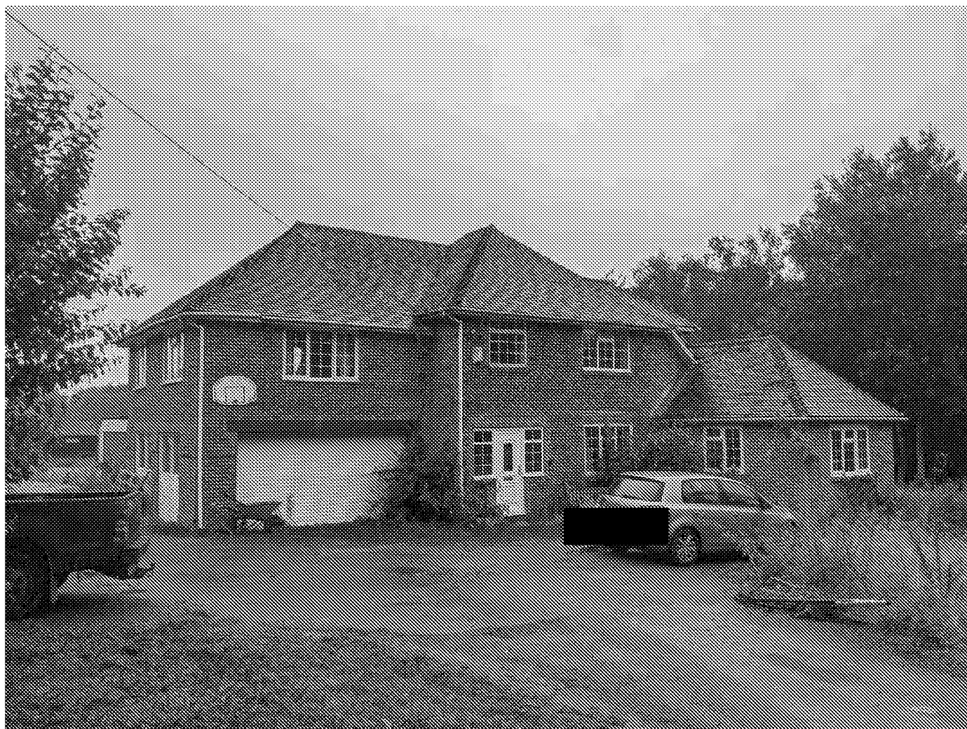
Photo 1 – View of the dwelling from the north-west.
