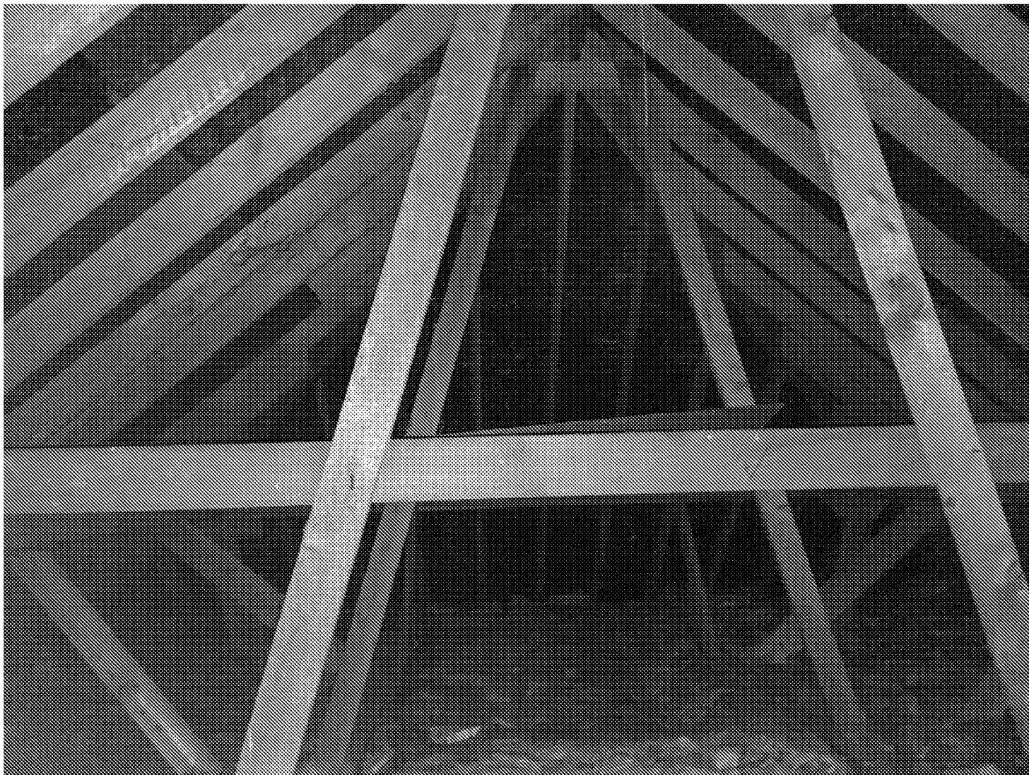
Photo 3 – View of the loft of B1.
