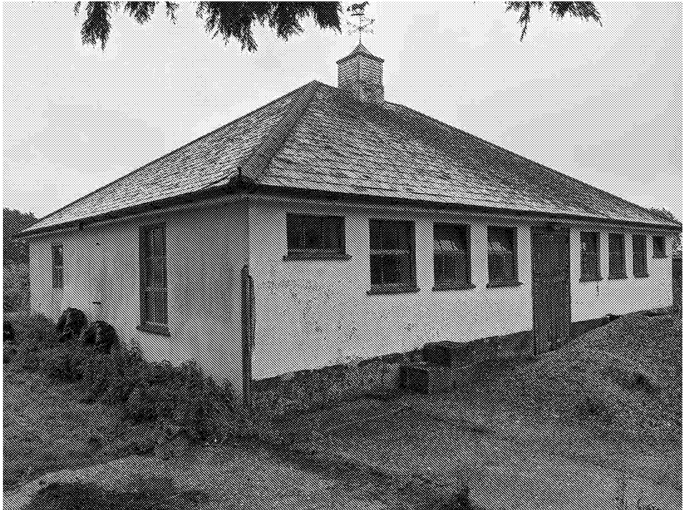
Photo 6 - The building B2, viewed from the north-west.
