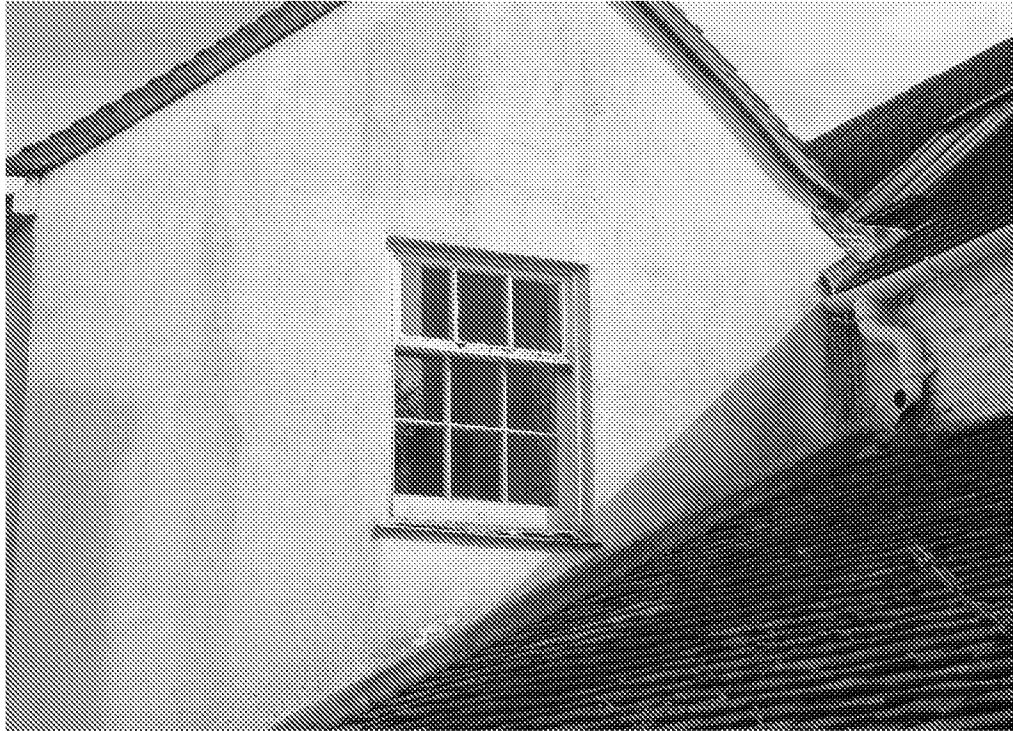
First Floor – Western Elevation Window FW2
