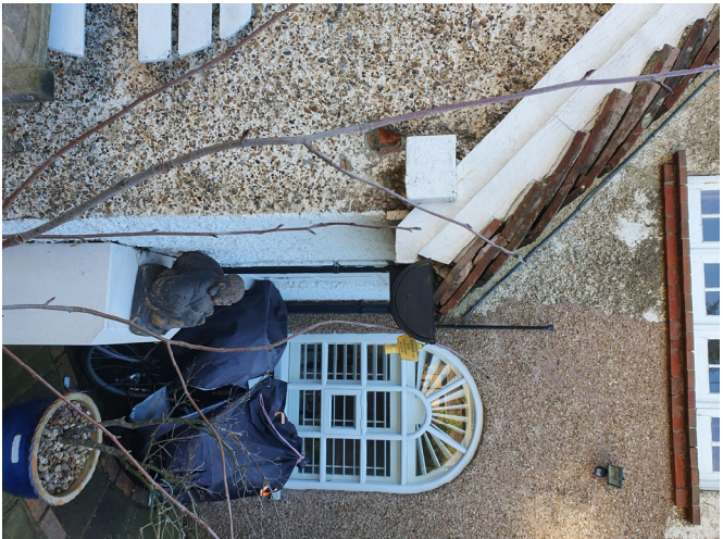
North Elevation(Side) Photo 6
