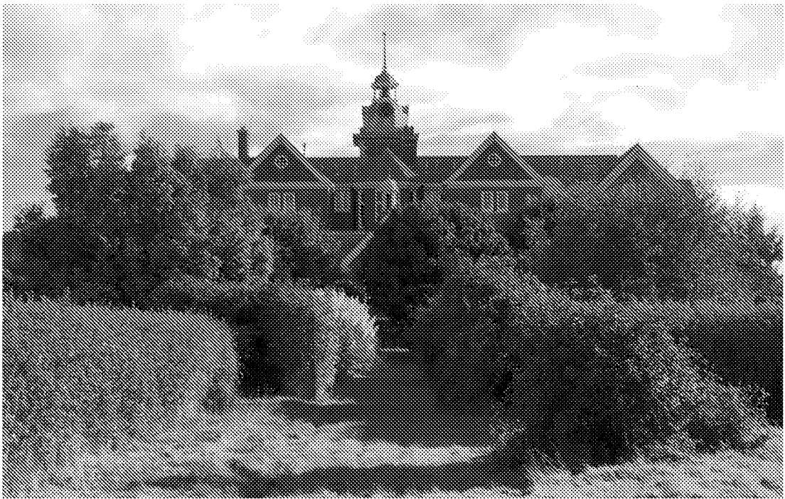
FIG . 17 - PBA PHOTO - NORTH ELEVATION OF THE CONVALESCENT HOME
