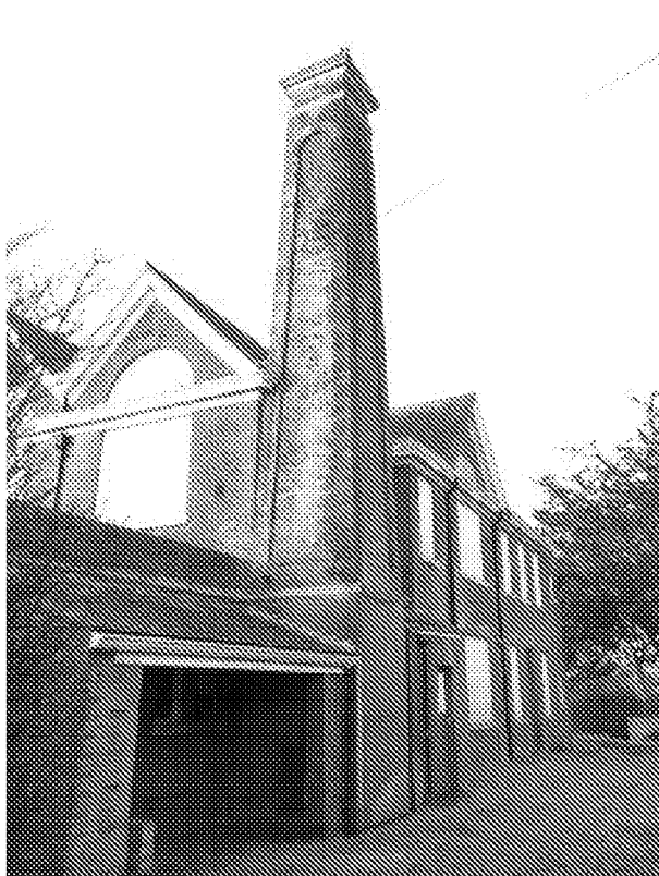
FIG. 21 - PBA PHOTO - LAUNDRY NORTH-EAST CORNER
