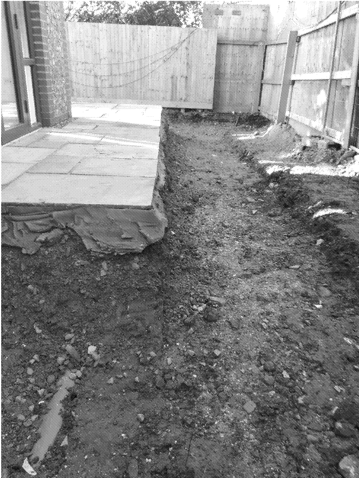
Figure 16 – Area of impacted soils in west of site excavated to 600mm below finished levels prior to soil placement.
