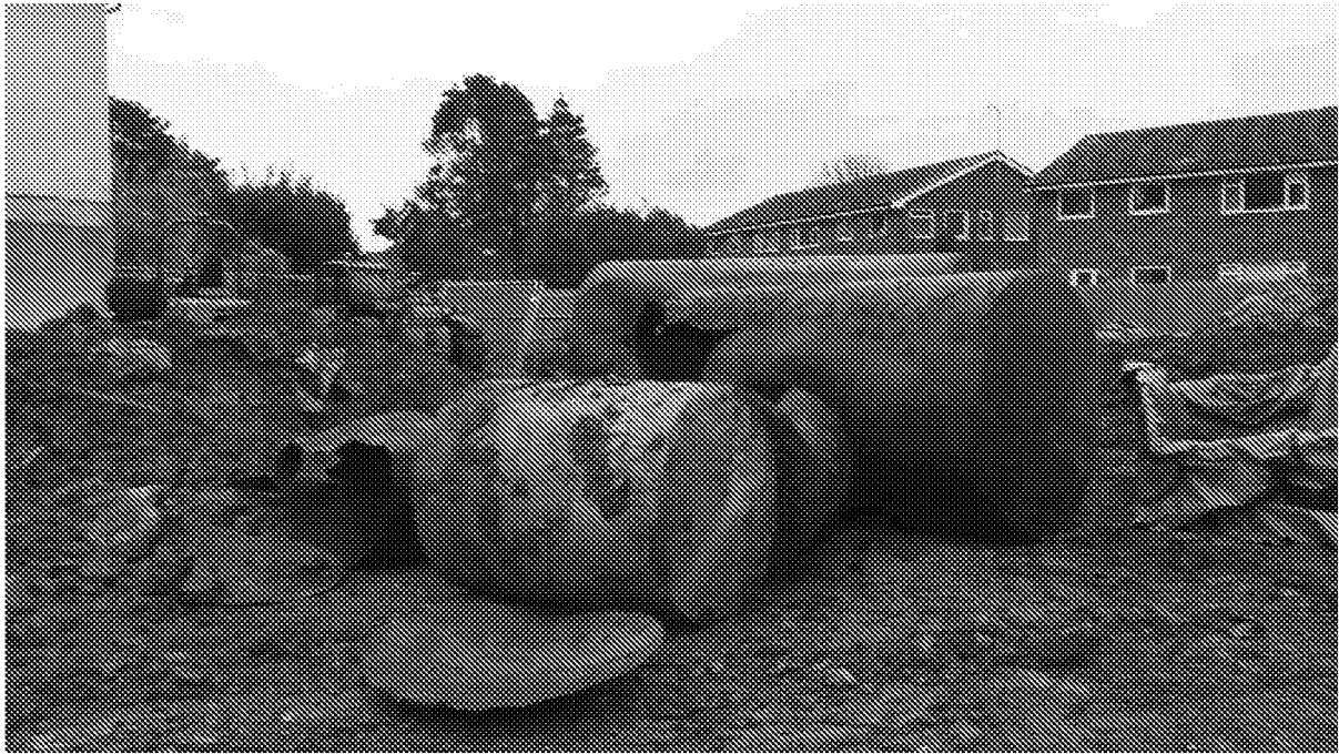
Figure 8 - Former fuel tanks following gas free and removal from source location
