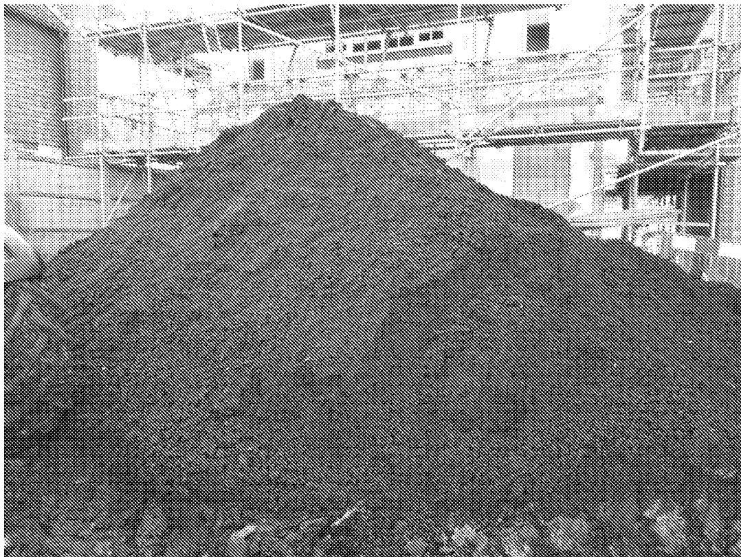
Figure 13 – Imported topsoil stockpile 2, sampled by REC on 20/02/2019
