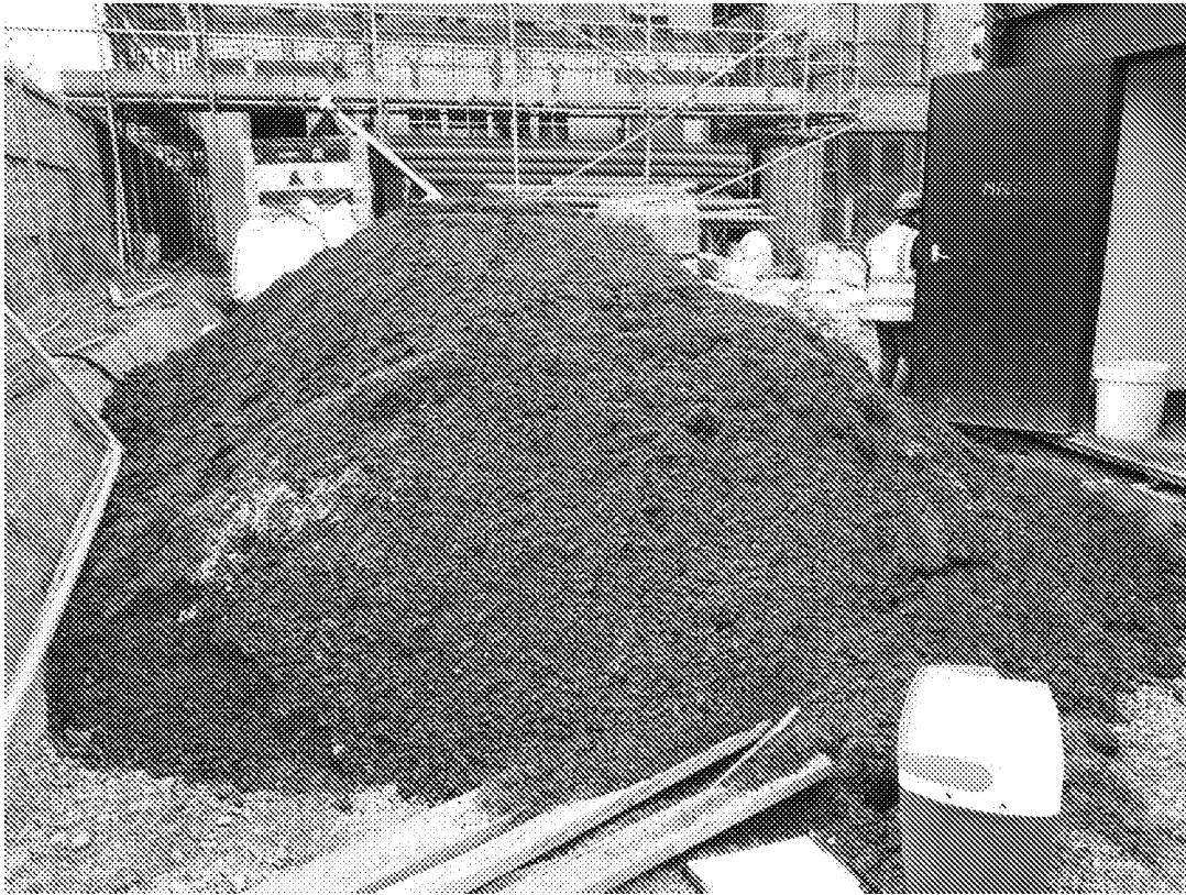
Figure 14 – Imported topsoil stockpile 4, sampled by REC on 21/03/2019
