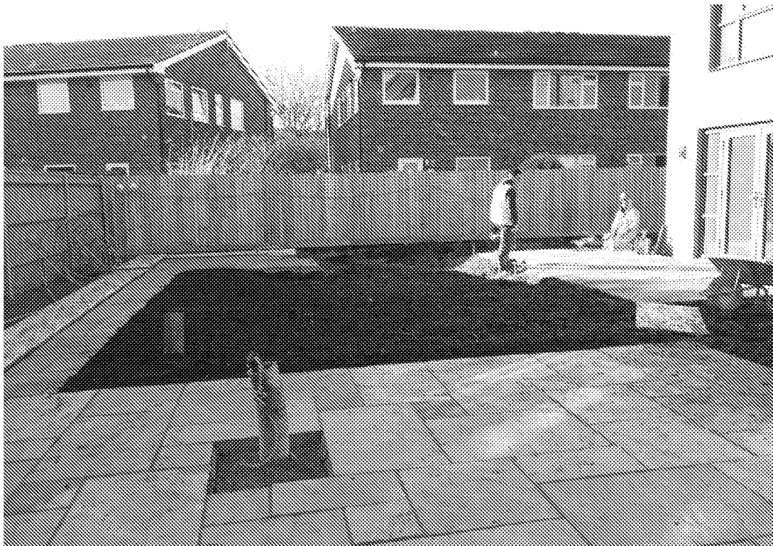
Figure 15 – Imported soil placed in communal gardens in southeast corner of site. Groundwater monitoring wells remain exposed prior to setting beneath flush covers.
