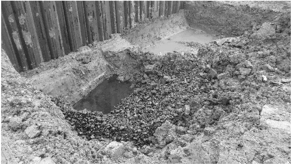
Figure 6 - Impacted materials within excavation in Southern Source area, groundwater at circa 7.0 mbgl. This excavation was made and subsequently backfilled prior to commencement of in situ remediation.
