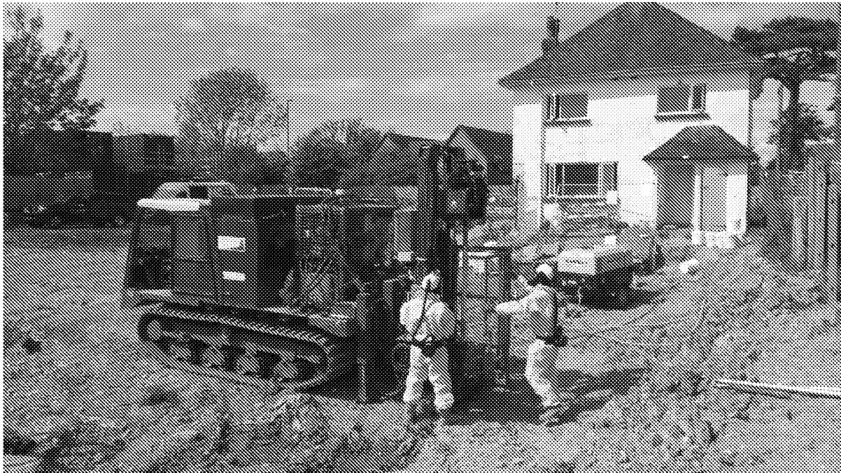
Figure 10 - During direct injection of oxidising agent into Southern Source area
