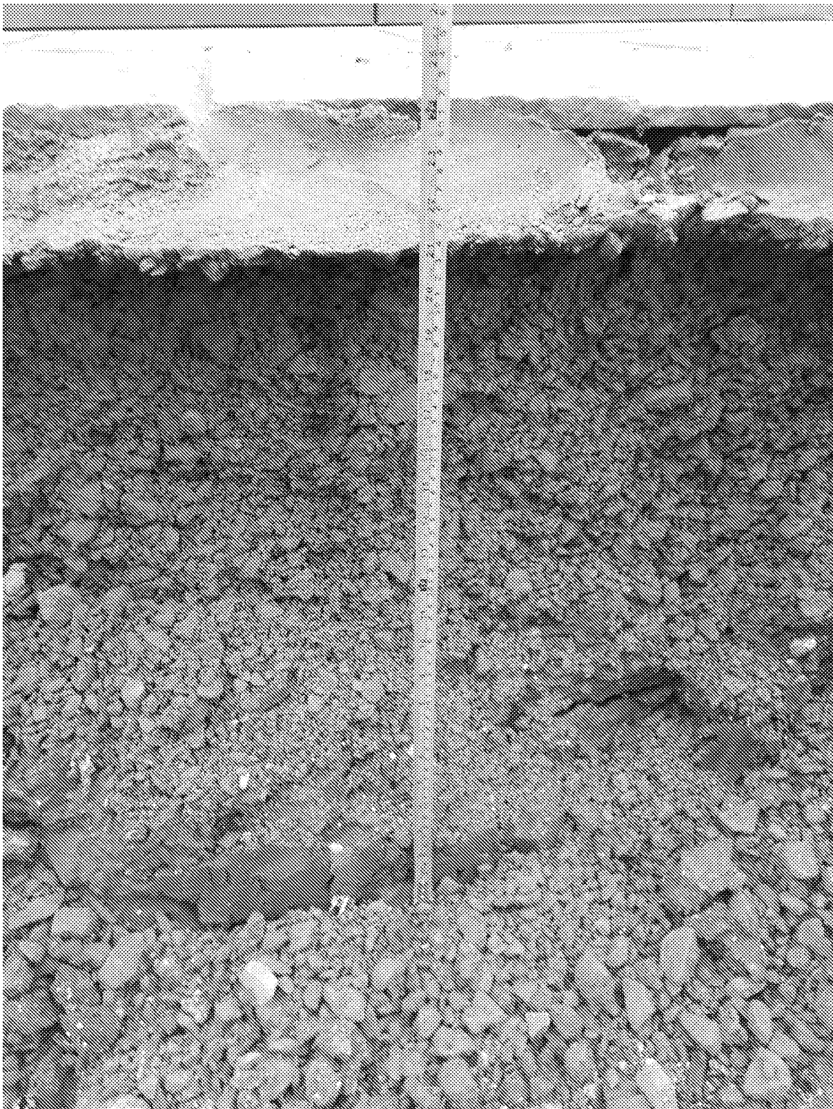
Figure 17 – Confirmation that 600mm depth has been achieved in west of site.
