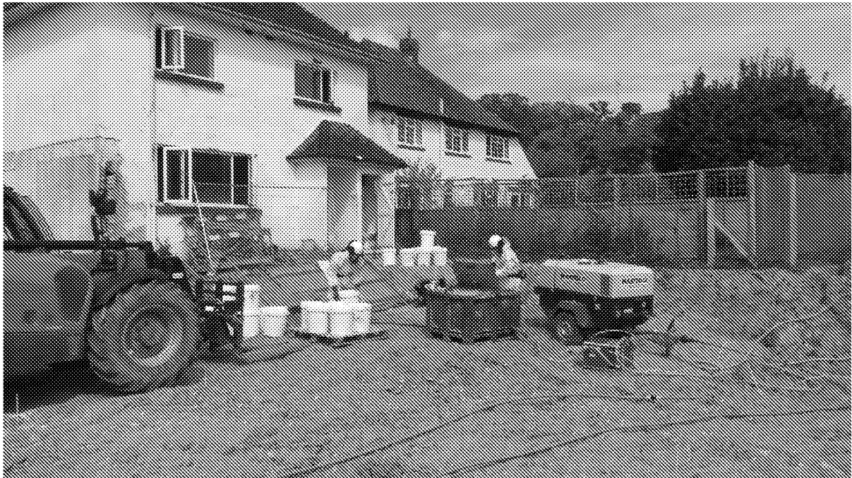
Figure 9 - Preparation of oxygen biochem for injection works (Tor Drilling engineers, operating on behalf of McAuliffe / Geostream)
