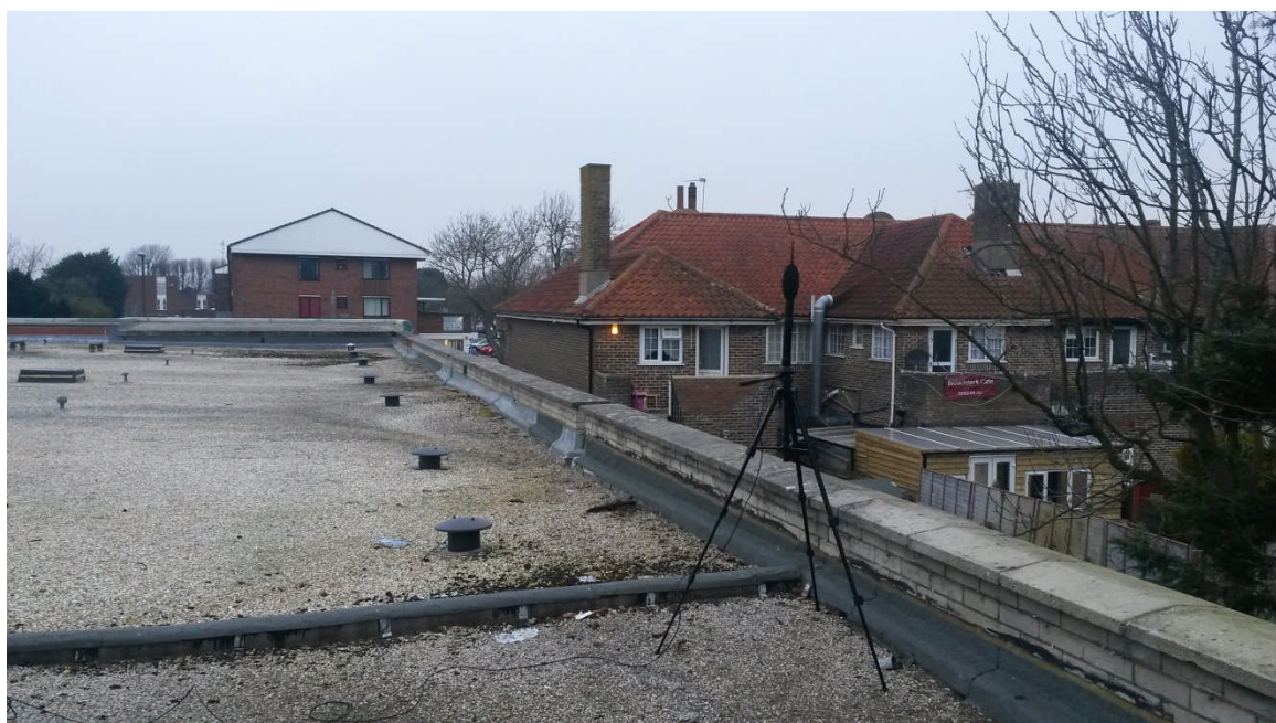
Photo 1 : Rear of residential dwellings above shops on Broadmark Lane
