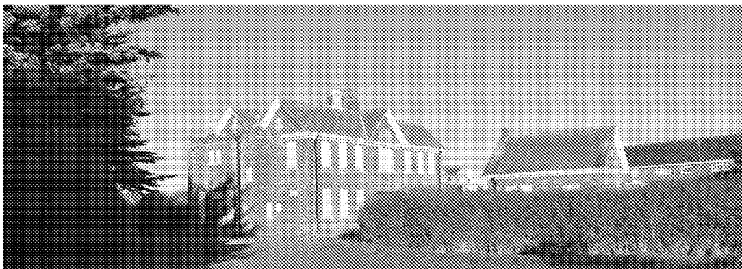
Figure 10: Western Elevation of the Laundry Block
