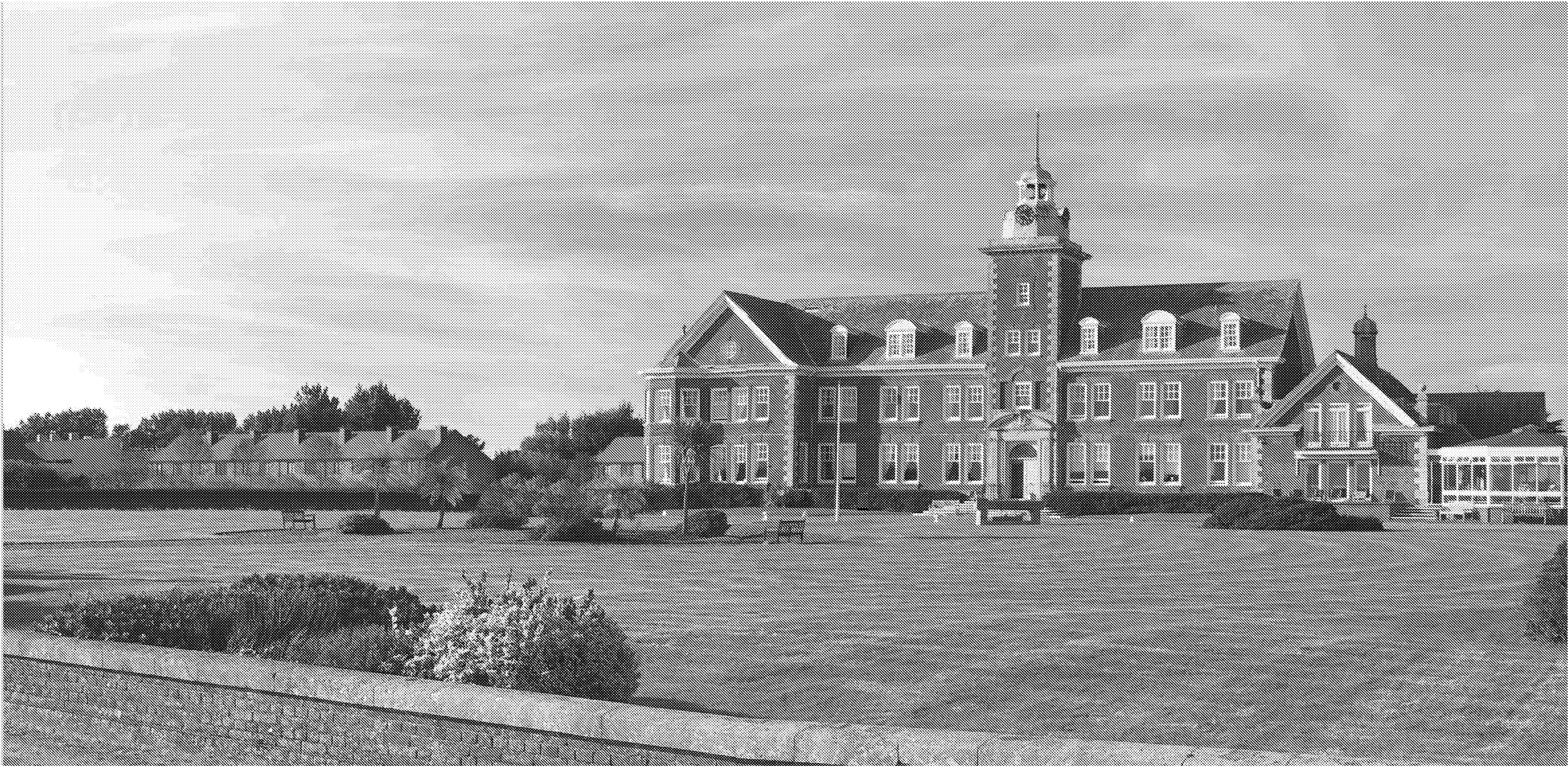
FIG . 89 - VIEW LOOKING NORTH-WEST FROM SEA ROAD WITH BLOCK A TO THE LEFT AND BLOCK B JUST VISIBLE BEYOND THE CONVALESCENT HOME
