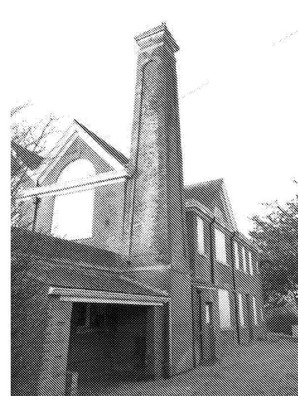
FIG. 21 - PBA PHOTO - LAUNDRY NORTH-EAST CORNER
