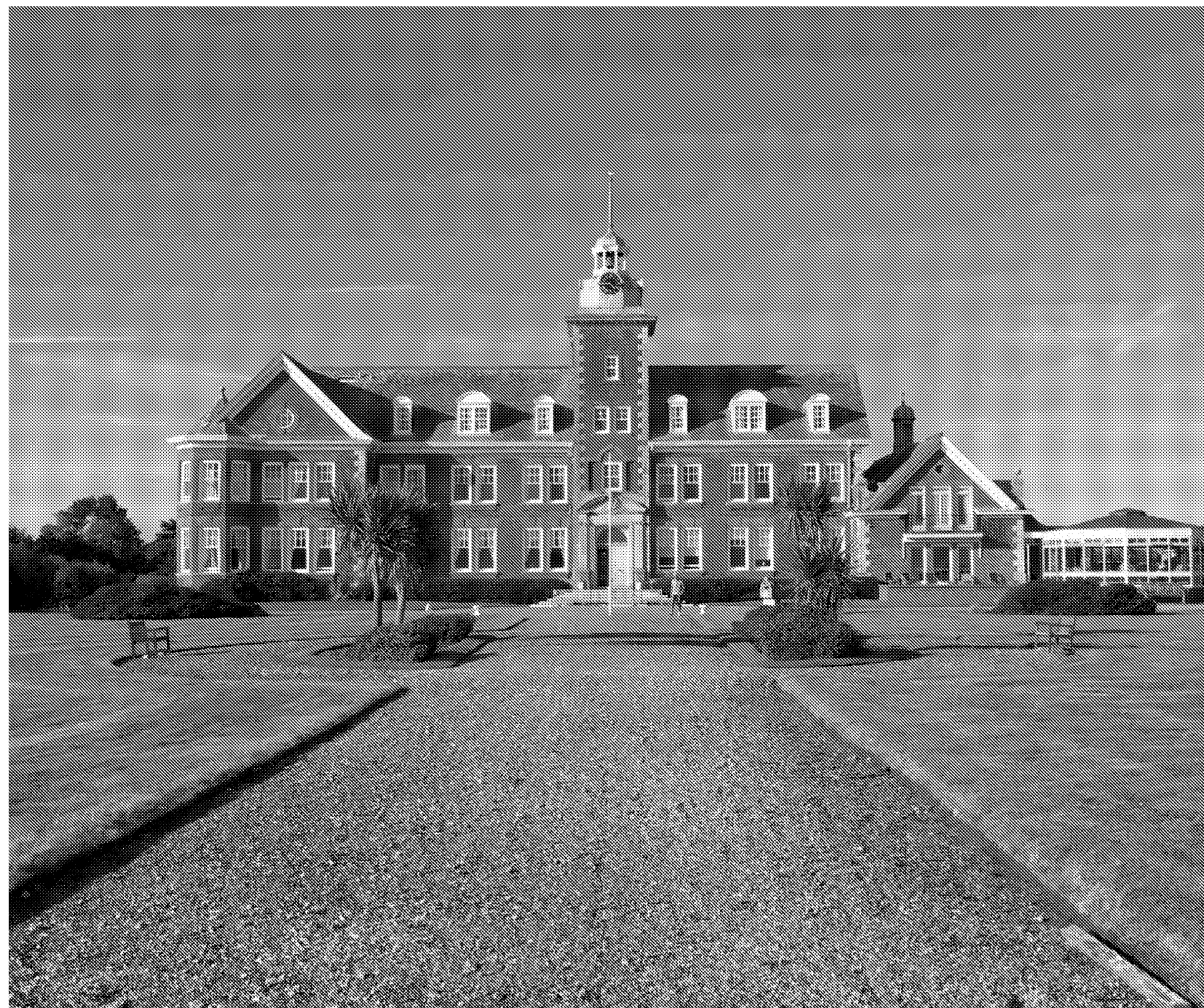
FIG. 1 - PBA PHOTO - THROUGH THE FRONT GATE - LOOKING NORTH TOWARDS THE CONVALESCENT HOME
