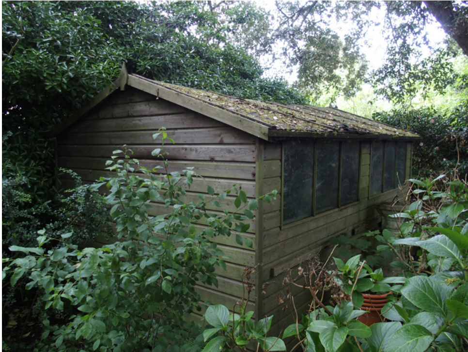
Photograph No. 13 - Southern shed to the south of the site (Building B2).
