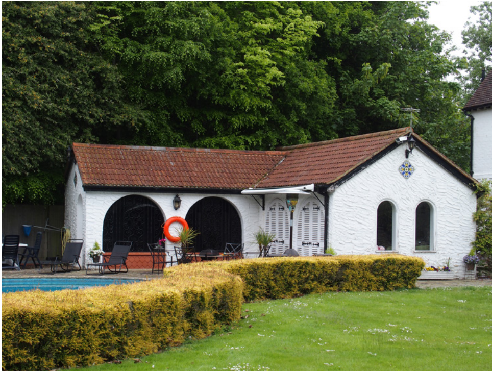
Photograph No. 15 - The pool house to the west of the site (Building B5).
