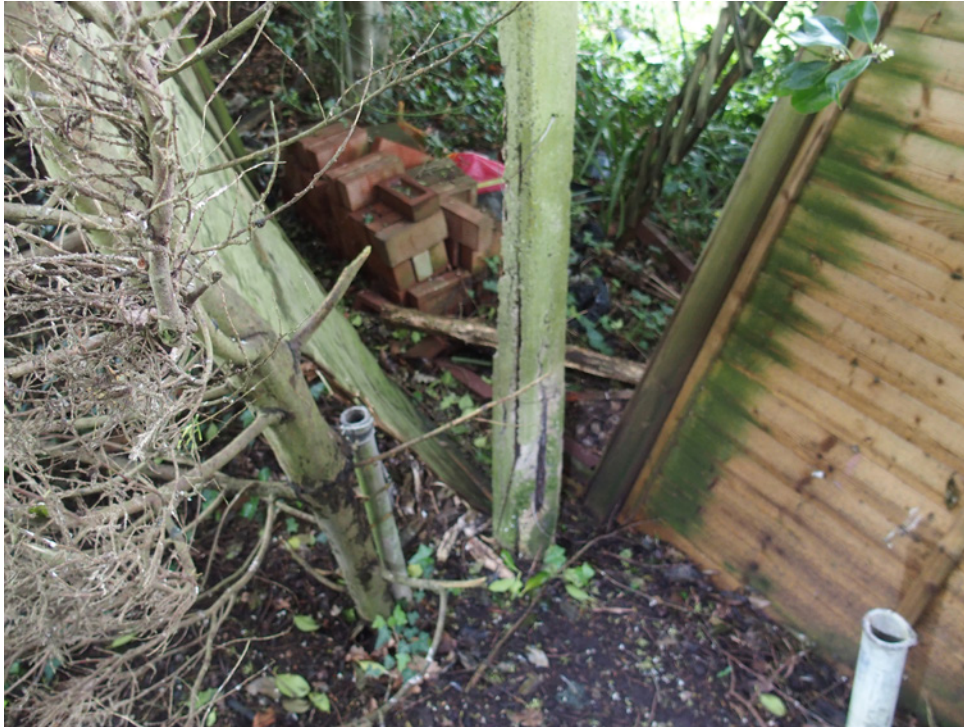
Photograph No. 11 - Collapsed fence to the north-west of site. A single hair indicative of badger was found here.
