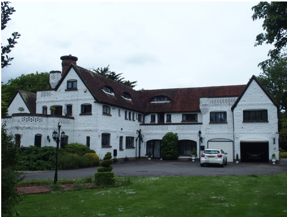
Photograph No. 16 - 'The Spires' main dwelling to the centre of the site (Building B6).
