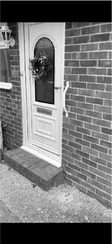
Existing stepped access
