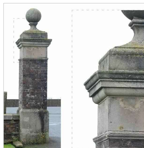
PHOTOGRAPH OF EXISTING PIER
