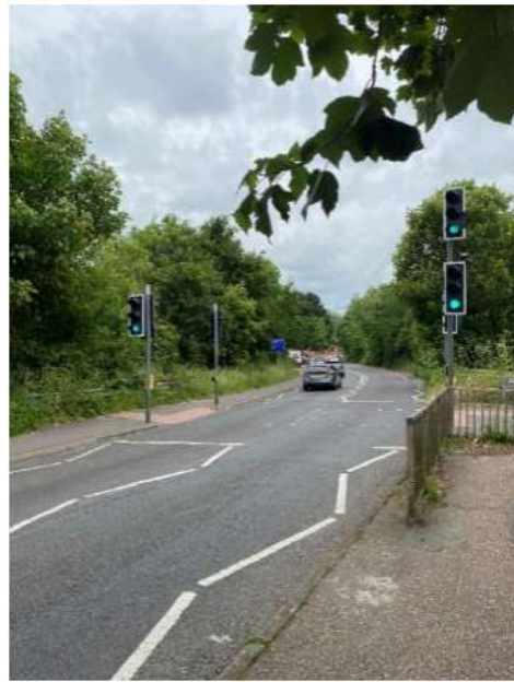
Photograph 6: Signalised Pedestrian Crossing (Mill Lane)
