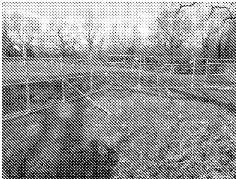
Example of Heras fencing
