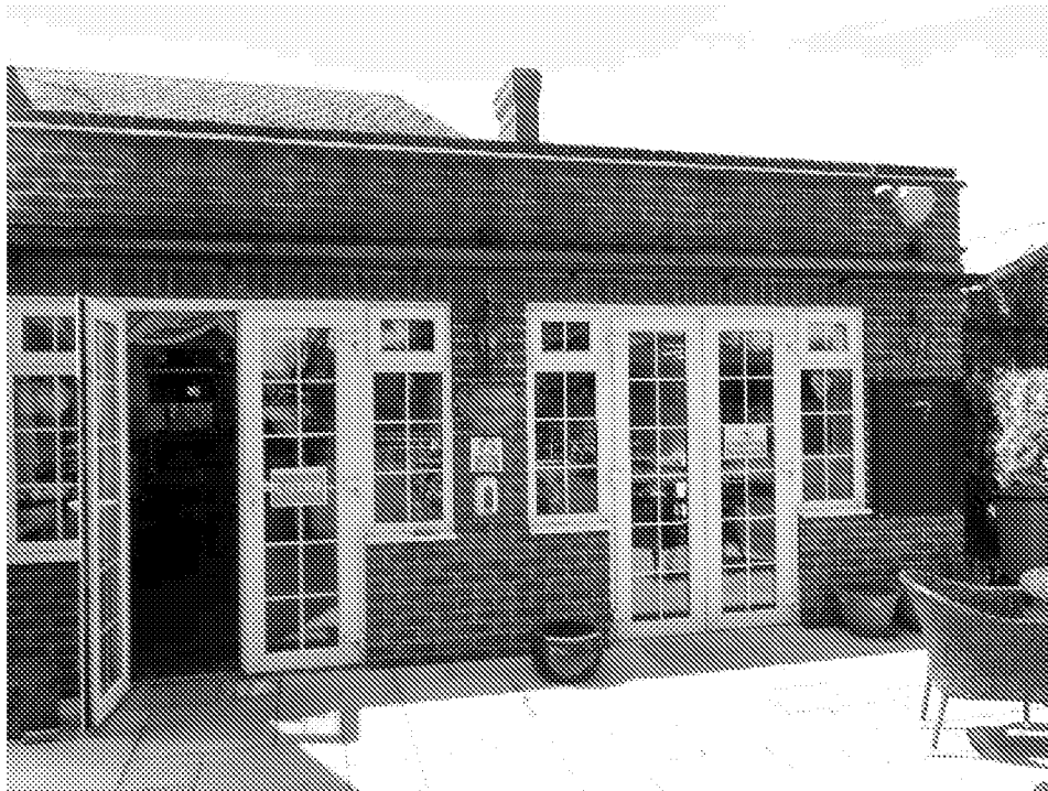
4 – Eastern side of rear extension
