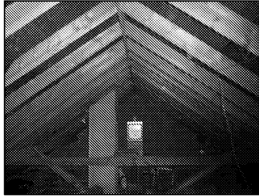
Figure 7 Roof void, No.2 Broadmark Lane
