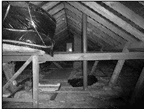
Figure 12. No.18 Vernon Close, roof void.
