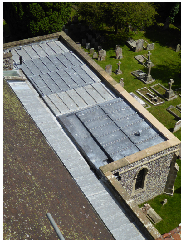
photo of south aisle and vestry roofs as existing
