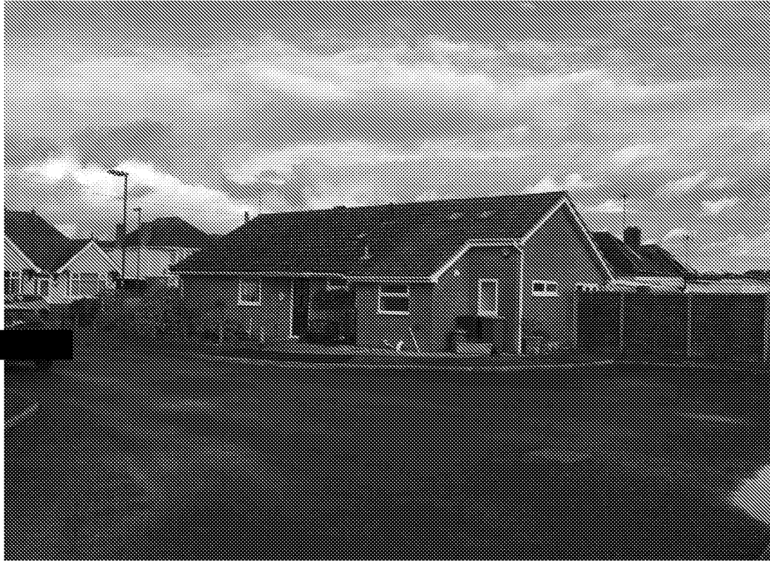
VIEW OF FRONT PRINCIPLE ELEVATION AFTER COMPLETION OF EXTENSION REPLACING THE ORIGINAL GARAGE
