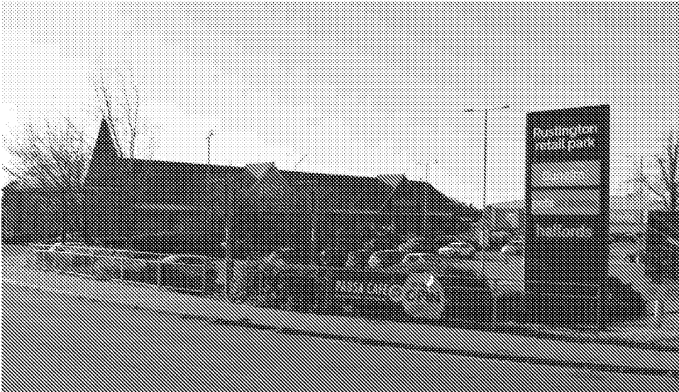
3. View looking south-west from slip road off A259 towards Rustington Retail Park
