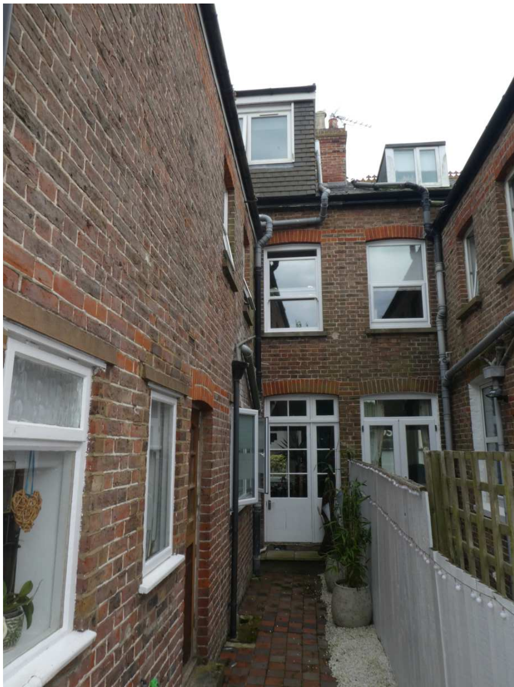
EXTERNAL REAR PHOTO SHOWING SIDE RETURN
