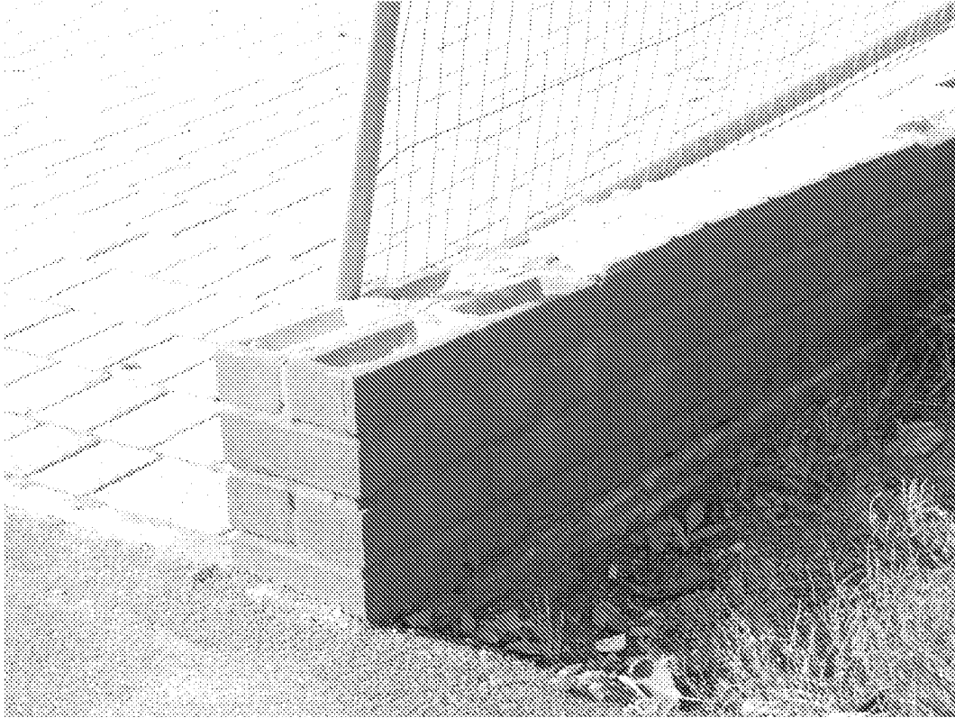
Front access, original brick edging details visible under new brickwork (to be removed)
