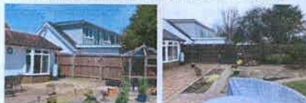
Rear elevation looking north
