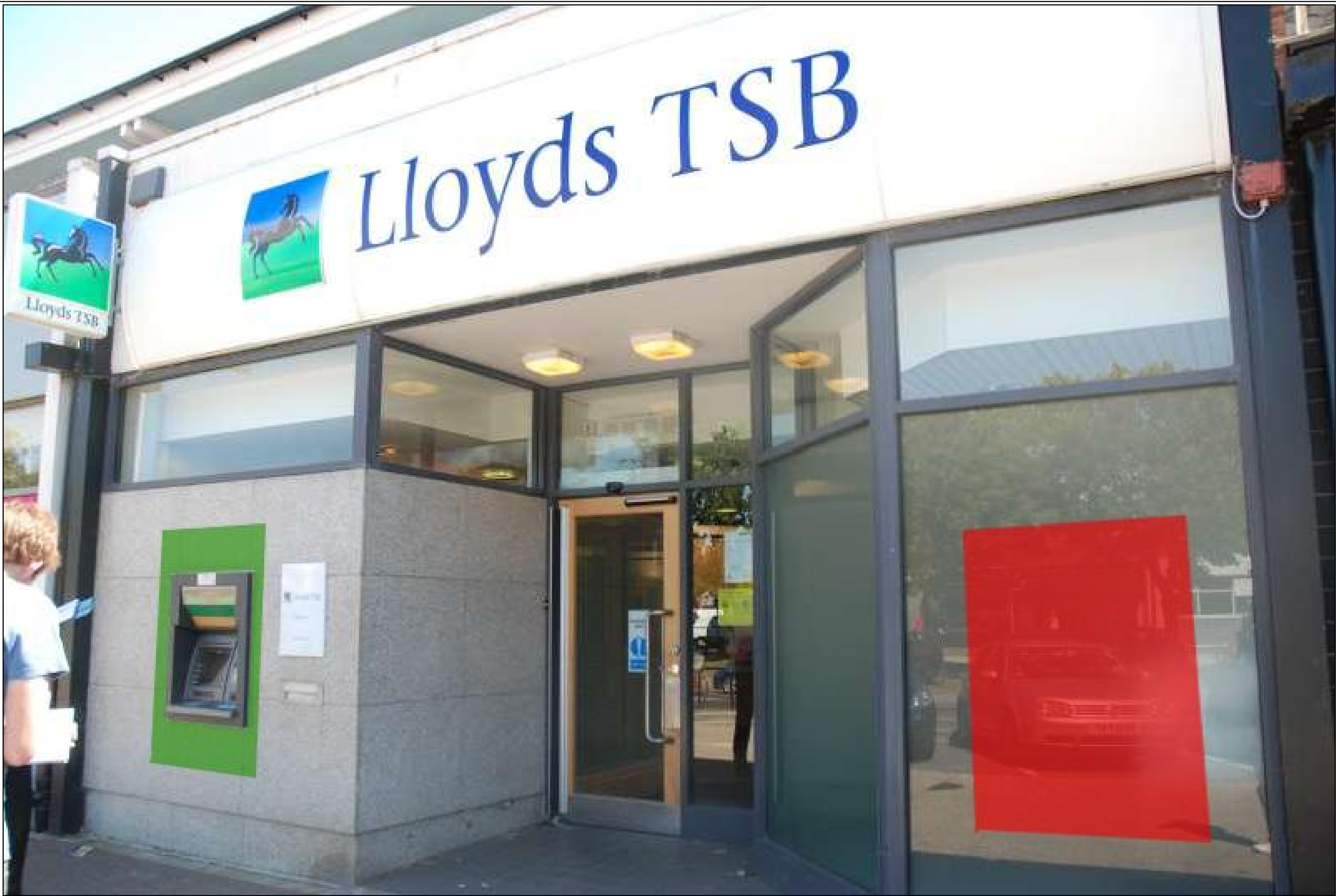
Photographs of Effected Elevations – N.T.S
